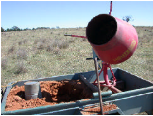
Figure 3. A cement mixer was used to thoroughly mix diluted chemical and soil.
