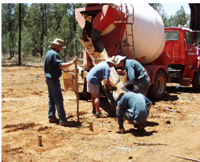
Figure 17. Treated soil was placed into holes directly from the cement truck.
