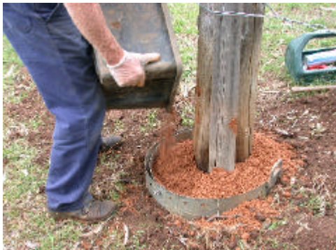
Figure 5. Chemically treated soil was placed between the cowling and the pole.
