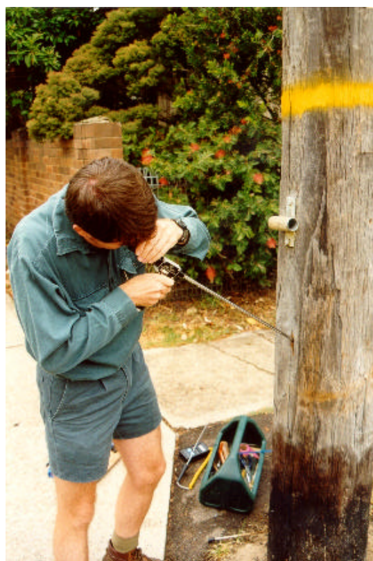
Figure 12. A borescope was used for inspecting internal voids for termites.
