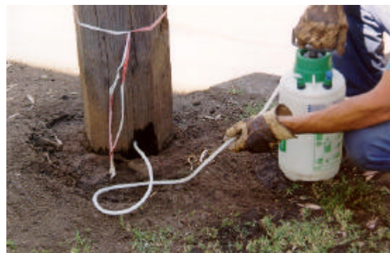
Figure 7. Chemical mixture was injected into poles with internal voids.
