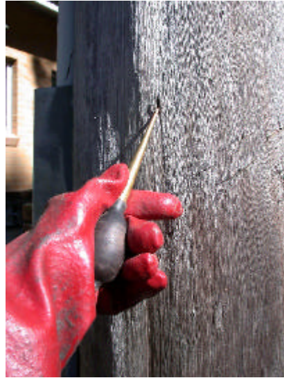
Figure 8. Dust is puffed into a check using a standard pest control industry hand applicator.
