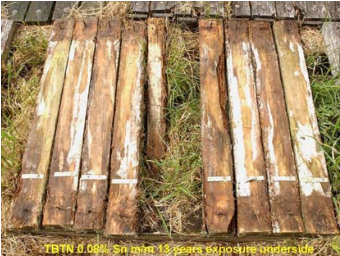
Figure 3. TBTN-treated P. radiata decking with 0.08% m/m tin after 13 years, underside.
