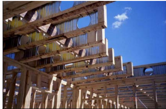
An LVL strongback has been run through the web holes of these cantilevered T30 joists that form a curved stairway void, to dampen live load vibration. Note the double web stiffeners fitted to the end of a joist that finishes at a web hole.
