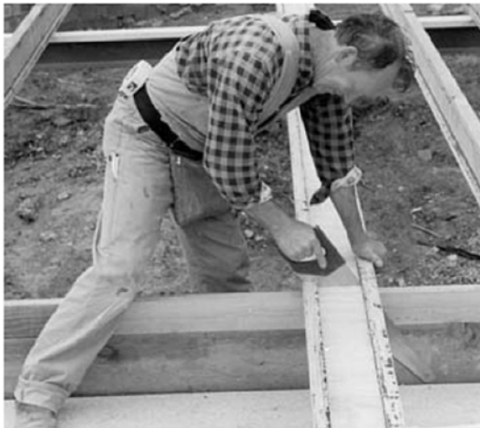
Hybeam engineered timber joists can be readily docked to length on site.
