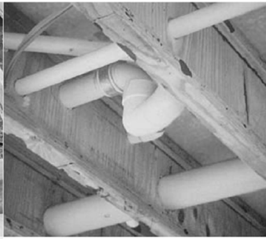
Easier installation of plumbing and electrical services within the floor depth.
