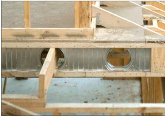
A 190x4577 strongback passes through T30 double joists, to share upper level tile roof & non-masonry parallel wall loads with the stud wall below on one side, and with the adjoining TECBEAM joists on the other.
