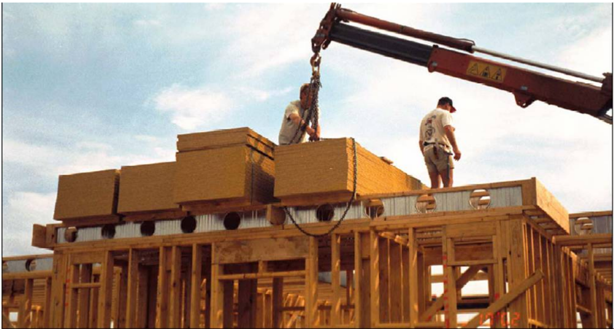
T30-P910 joists at 450crs. spanning 5.8m easily support over four tonnes of sheet flooring during construction. These joists will spring back perfectly straight and undamaged once this flooring load is removed. TECBEAM's exceptionally high ductility means the joists can be relied on to take short term overloading up to double design load, without risk of collapse.
