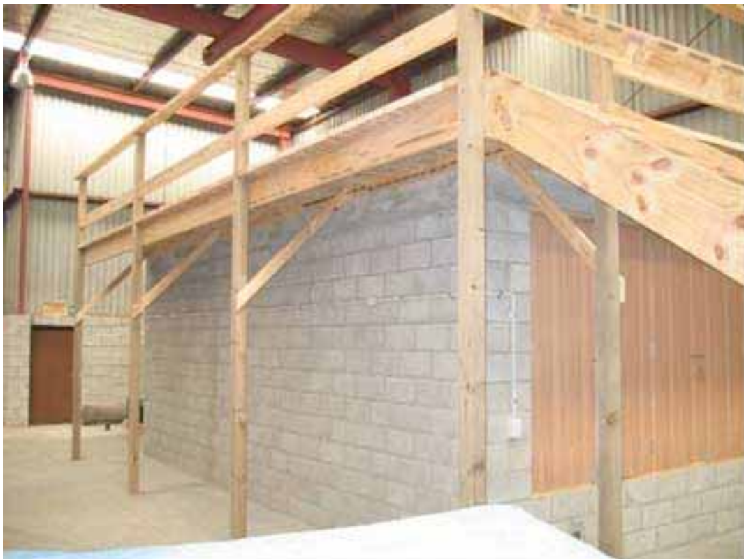
Figure 11-2. Side view of test chamber, showing entrance doors at right.
