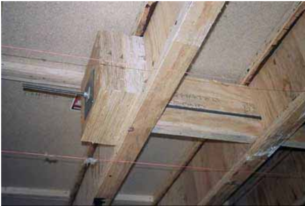
Floor 15. Ends of post tensioned beams
