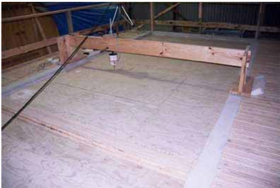
Floor 12. View of cross beam and plywood flooring from above
