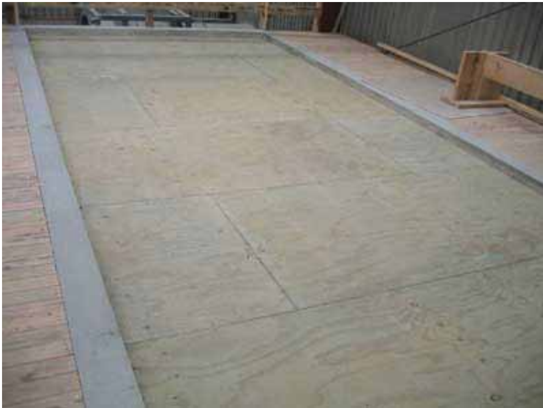
Floor 2. Overview of Plywood deck showing layout of plywood
