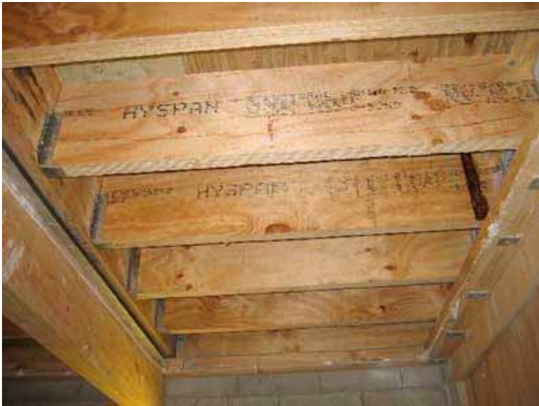
Floor 11. Underside of floor
