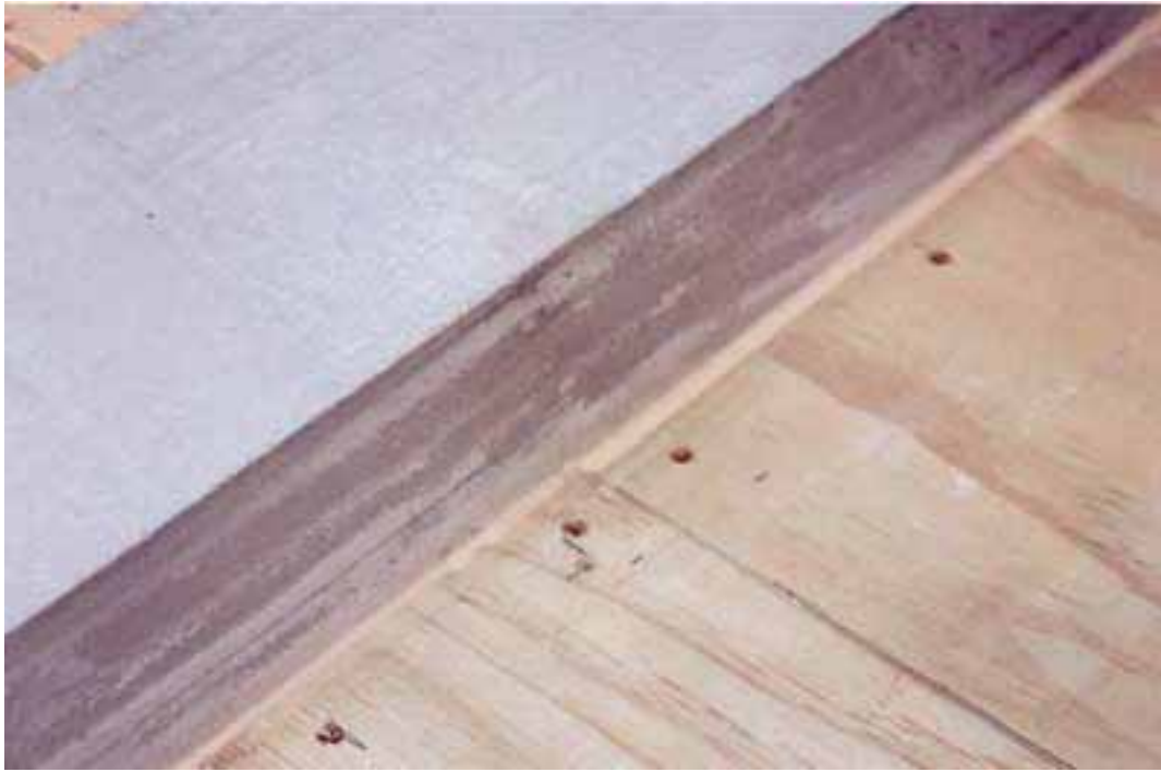
Floor 2. Edge junction between floor and test rig concrete beam
