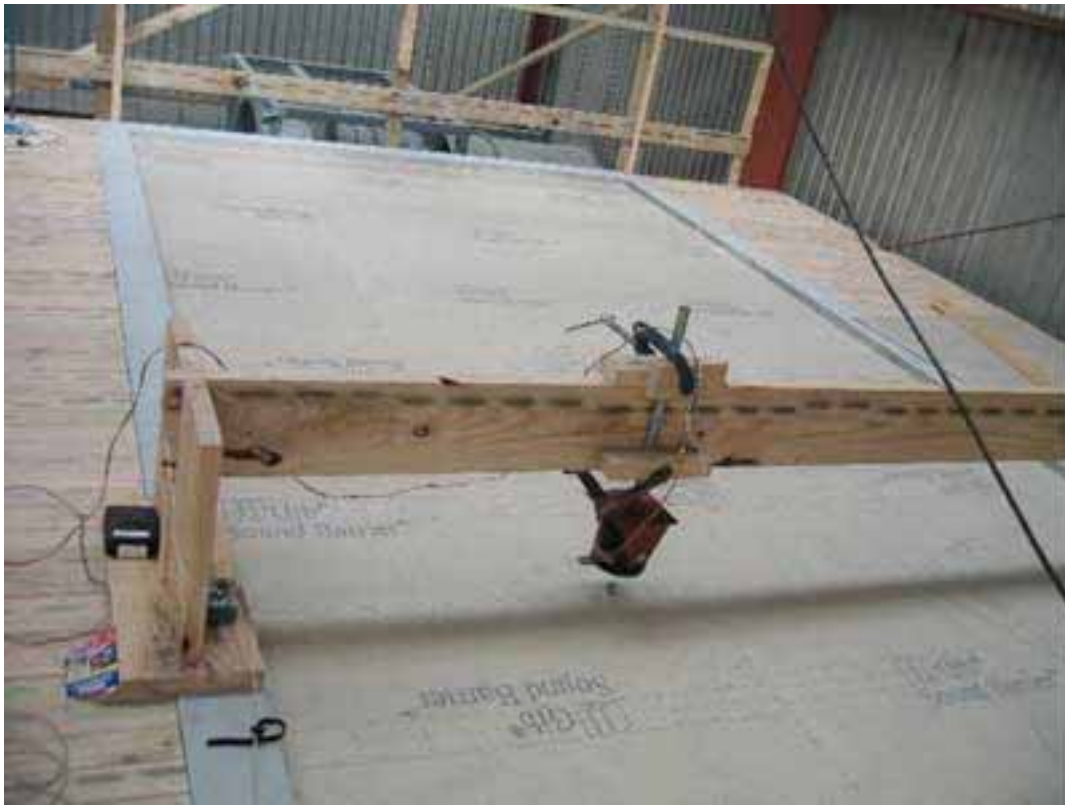
Floor 3. Overview of gypsum fibreboard deck showing layout.
