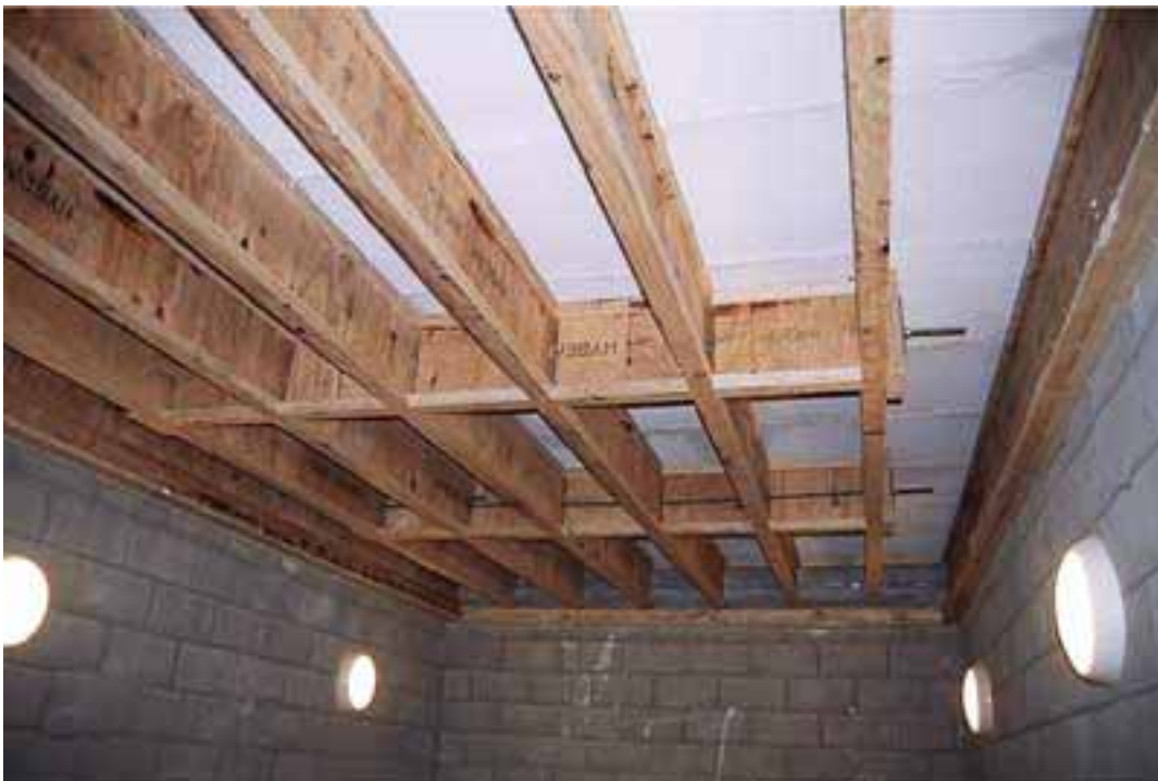
Floor 20. General view of the underside of the Hebel floor
