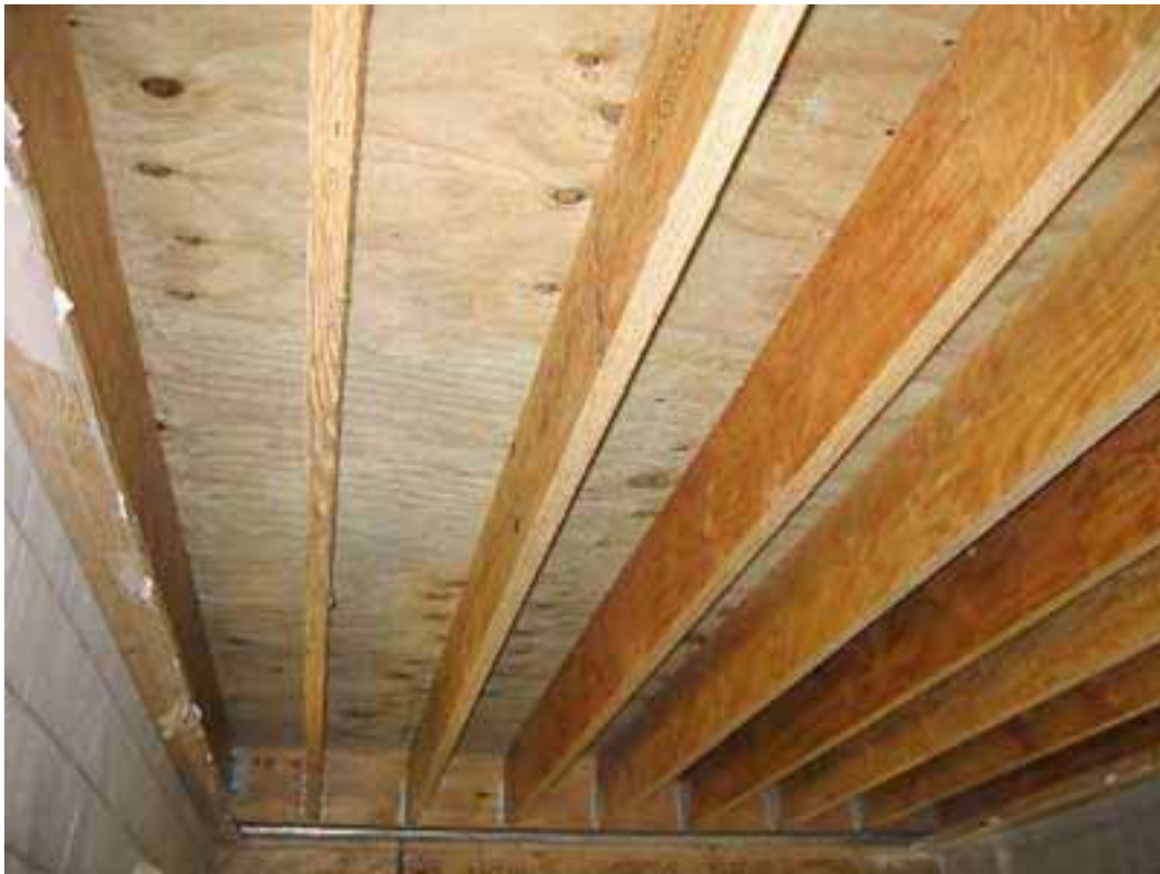
Floor 10. Underside of floor showing supporting beam at end.
