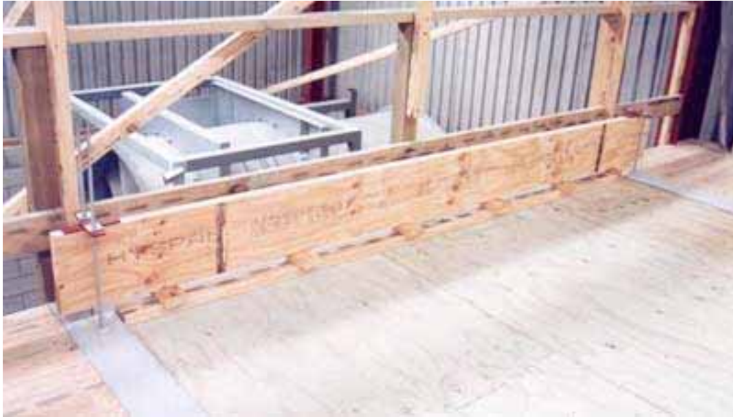
Floor 7. View of clamping down to end of floor
