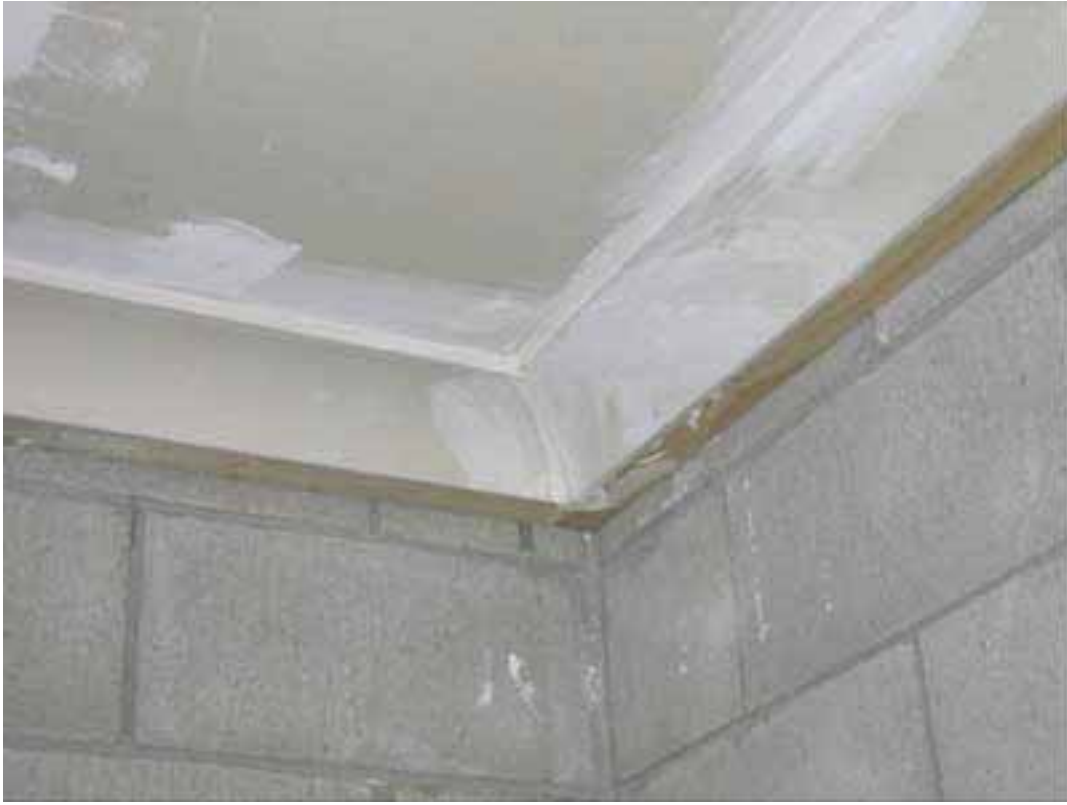
Floor 26. Coving in corner
