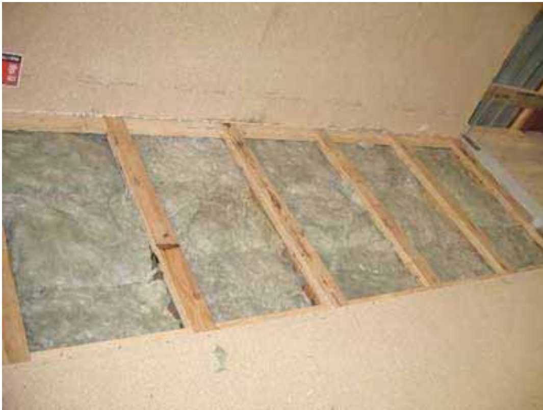
Floor 18: View of full cavities.
