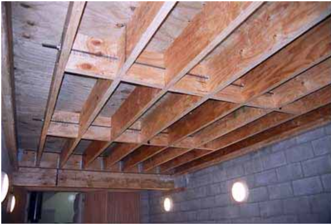
Floor 13. Illustrates two transverse beams under floor
