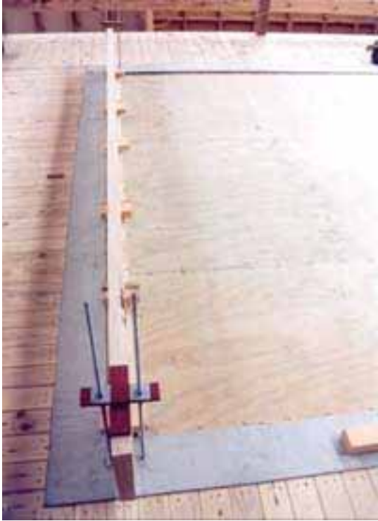
Floor 7. Clamping to ends of floor
