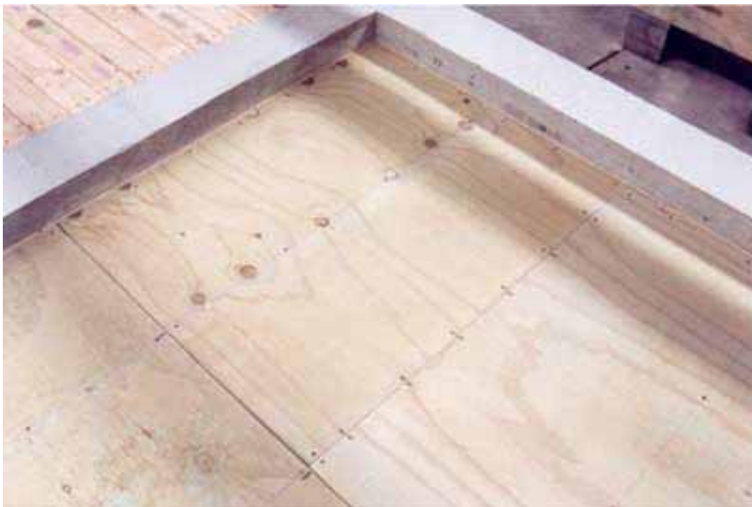
Floor 2. Plywood deck to reinforced concrete edge beam junction
