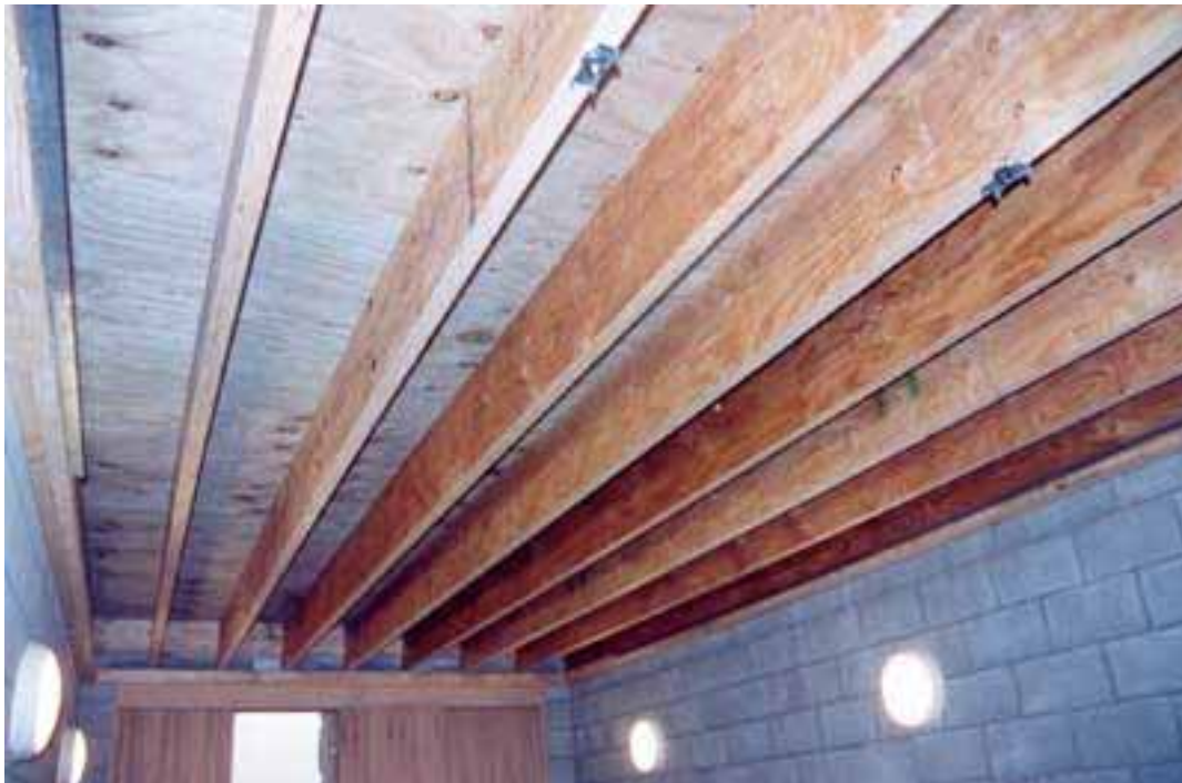
Floor 2. General view from below of 7m long 300x45 LVL joists
