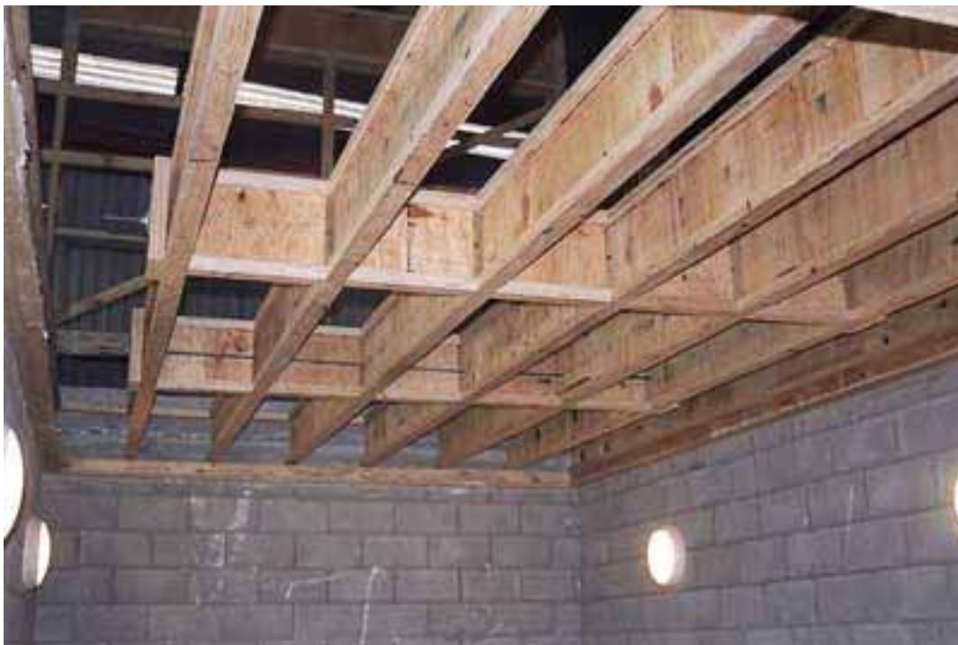
Floor 20. View of floor structure before Hebel flooring placed in position
