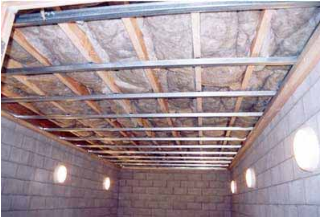
Floor 2. General view of ceiling system support
