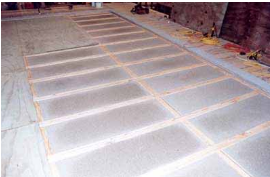
Floor 5. Sand infill between 45mm deep battens
