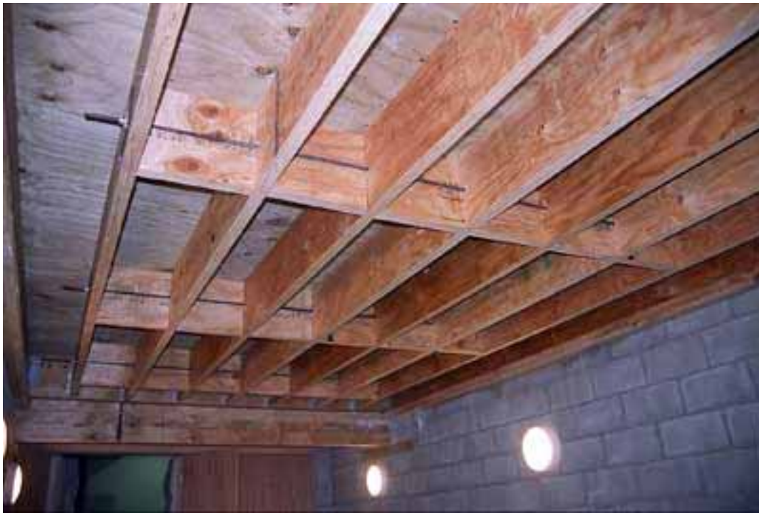
Floor 12. View of underside of floor showing four transverse stiffening beams
