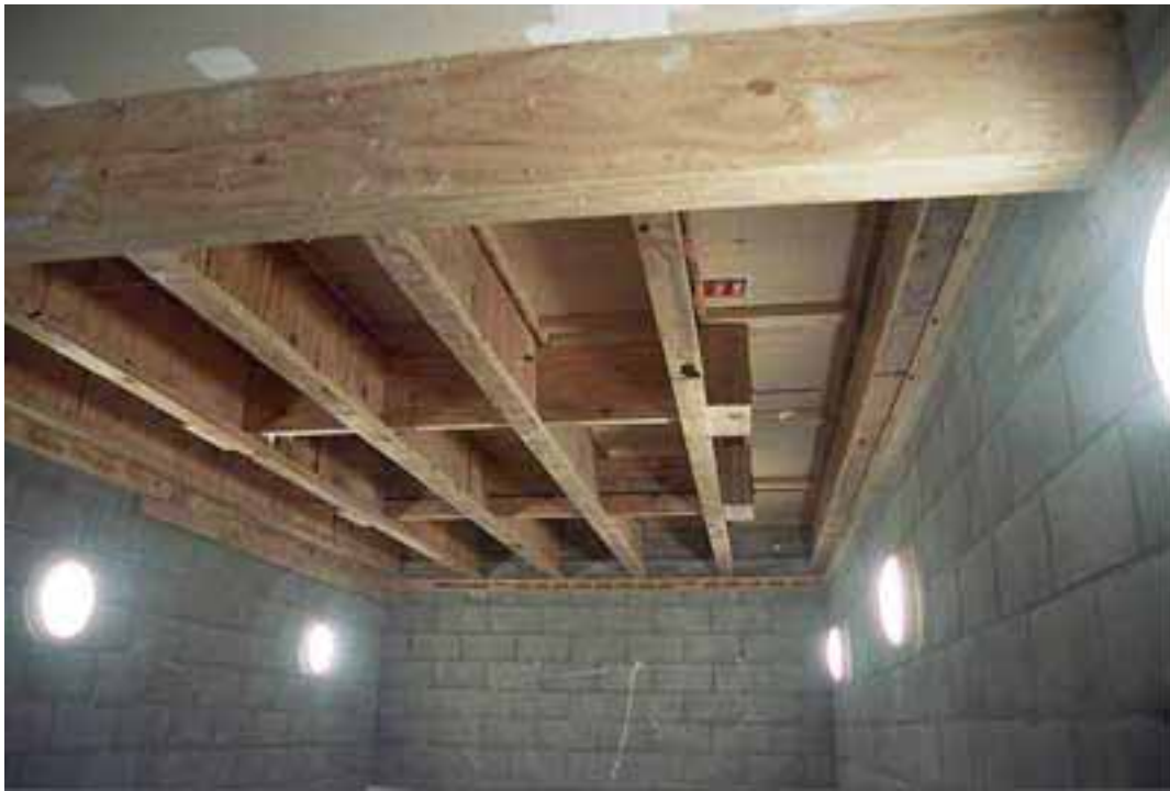
Floor 15. Shows 400 deep I joists at 600 centres with two central transverse beams up to penultimate joist
