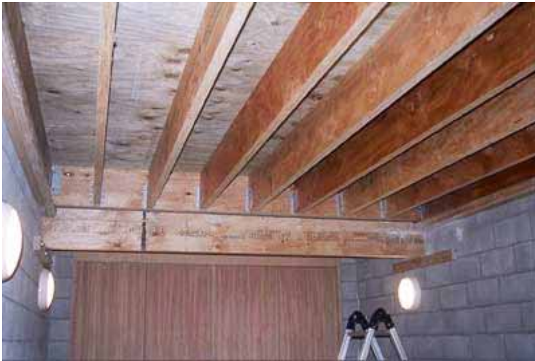
Floor 8. View of cross beam showing joist hangers
