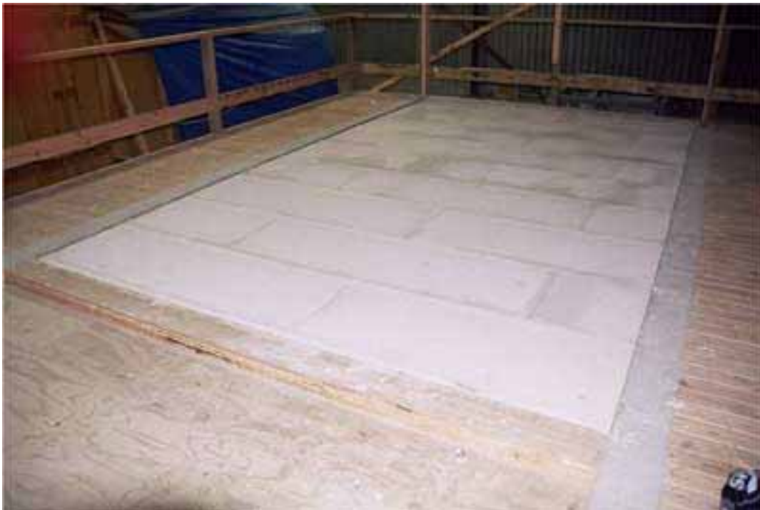
Floor 20. General view of the Hebel floor
