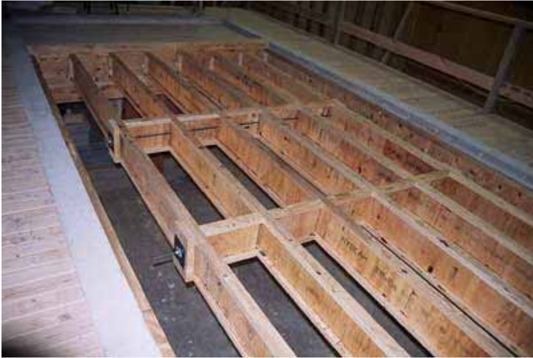
Floor 20. Close up view of the two transverse beams
