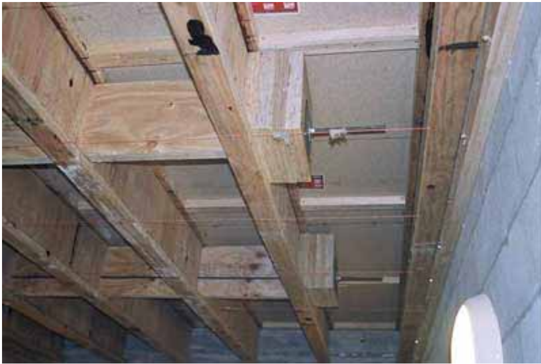
Floor 15. General view of the ends of the transverse beams
