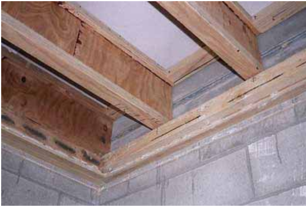
Floor 20. One end of joists simply supported on 100x50 timber ground off blockwork
