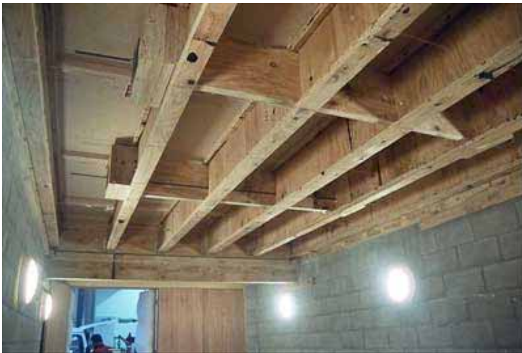
Floor 15. Shows 400 deep I joists at 600 centres with two central transverse beams up to penultimate joist
