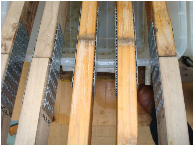
Figure 3.8 – Backout of non-coated joints in specimens A (plain finished)
