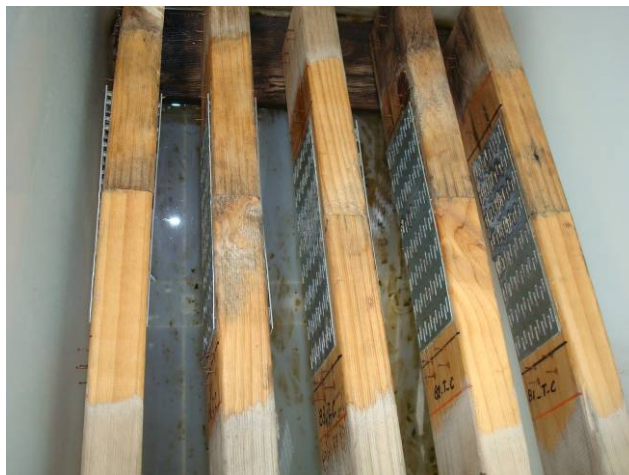
Figure 3.11 – Backout in joints coated with 'Seal and Peel' 660
