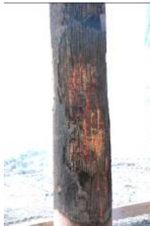
Figure 10 FireGuard CCA-treated radiata pine specimen one hour after testing at 60 kW/m 2 and being subjected to a 2 m/s wind
