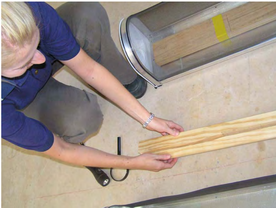
Figure 6: Opening and examining a split-beam in a living space (Photo: L Vagg)
