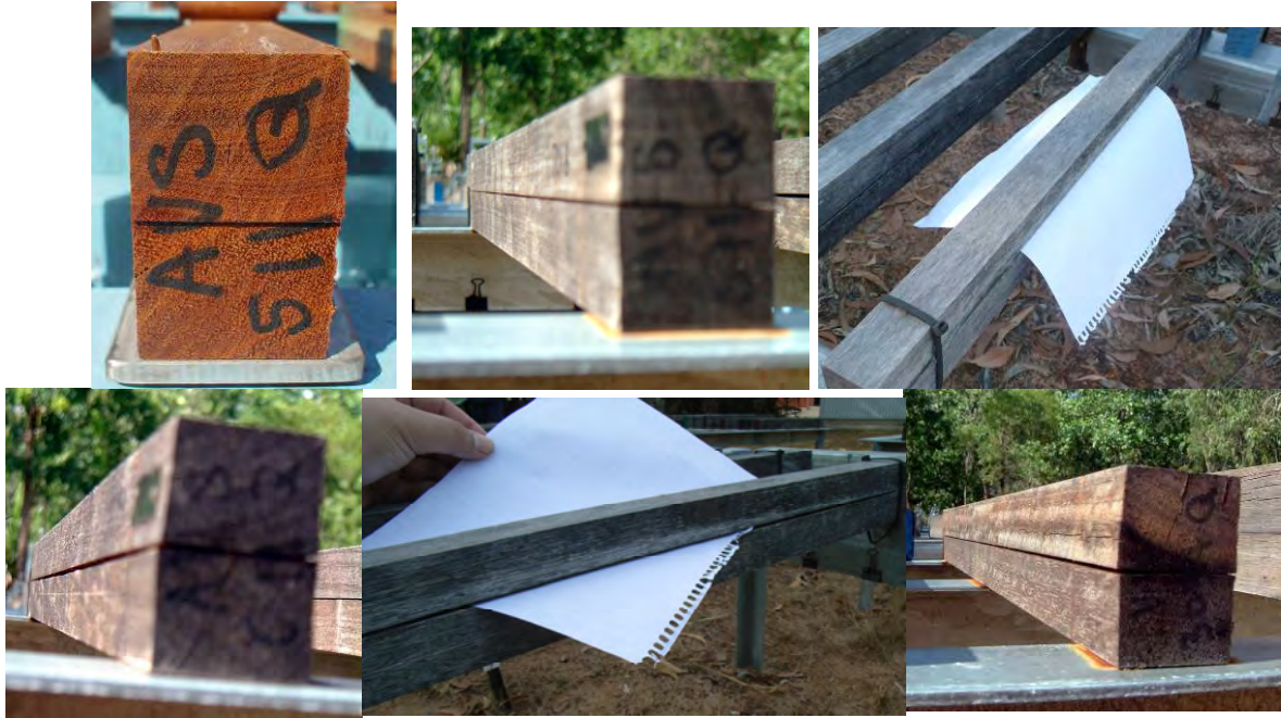
Figure 20. Some examples of the complete failure of non-loaded Spotted Gum samples in Darwin during the 3 year exposure test.
