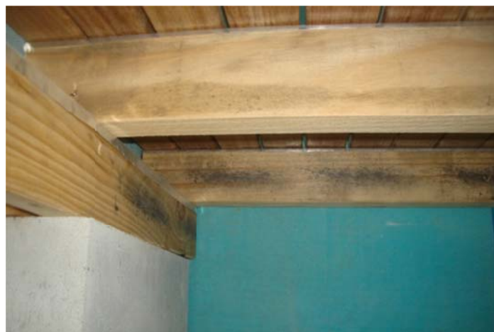
Figure 1 Metal flashing above timber joists
