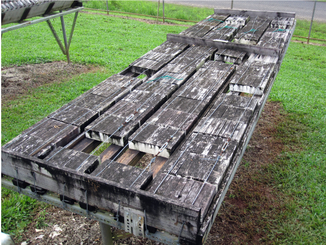
Figure 9. Frames 3 (near) and 4 (far) after 3.2 years at Innisfail with specimens laying horizontally (compare to Figure 2 when first installed). Blank positions held untreated controls that had crumbled due to decay.
