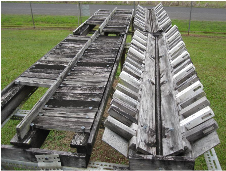
Figure 48. Raised deck (left) and embedded test (right) at Innisfail after four years.
