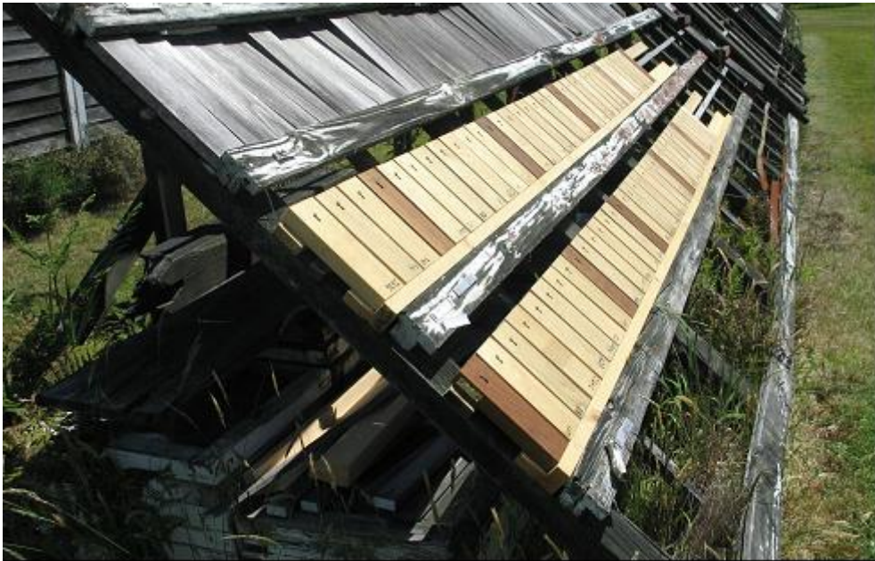
Figure 6. Flat panel test installed at Rotorua.
