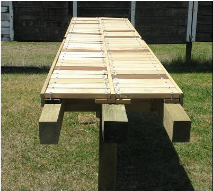
Figure 13. Raised deck installed at Rotorua.
