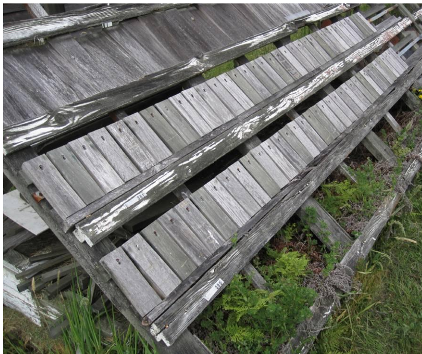
Figure 42. Flat panel test at Rotorua after four years.
