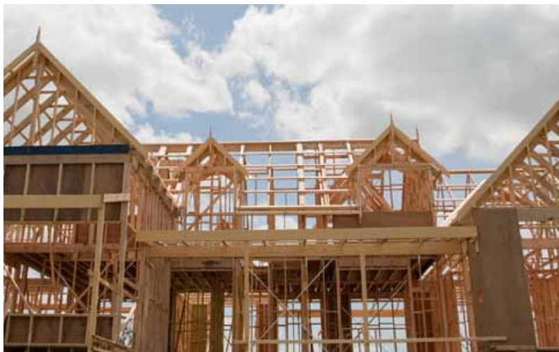
Construction of a house in the Yarra Valley, Victoria, using a timber frame
