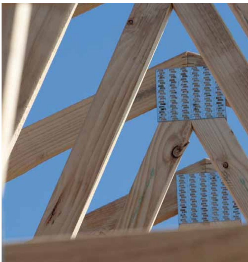
Nailplate apex joints in timber roof joists
