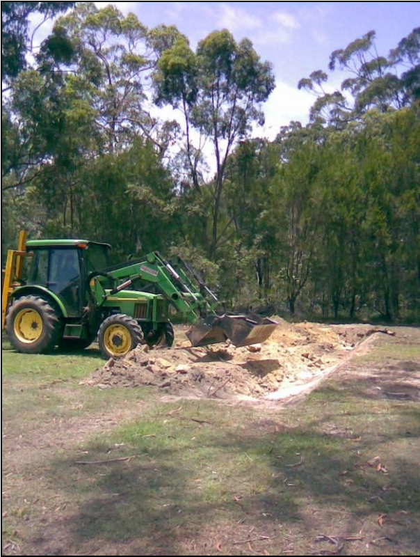
Figure 15 Digging the trench
