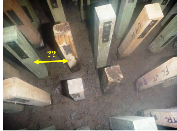
Figure 43 Saturated stake between adjacent dry stakes
