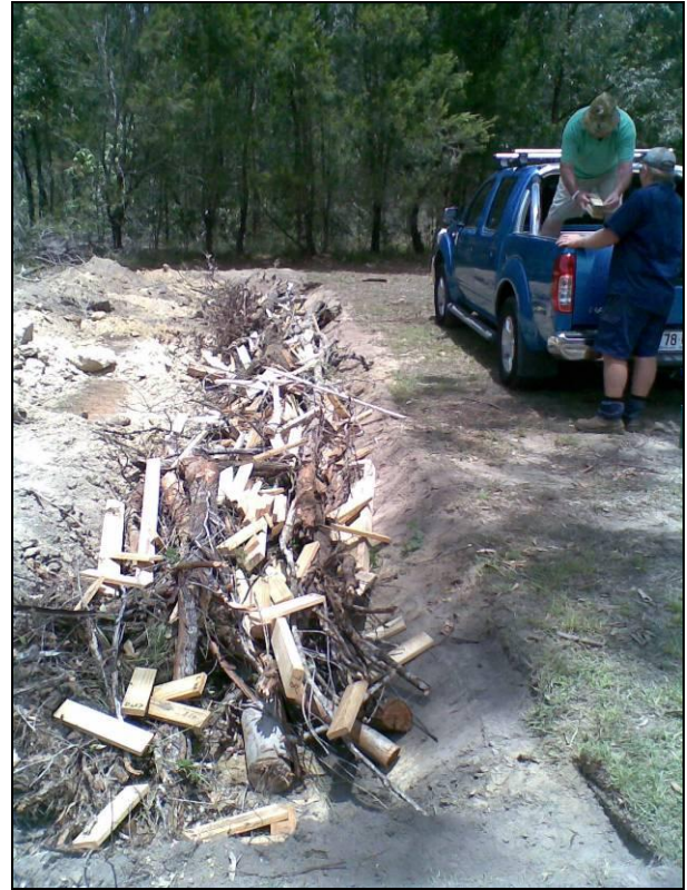
Figure 16 Filling the trench with softwood and hardwood
