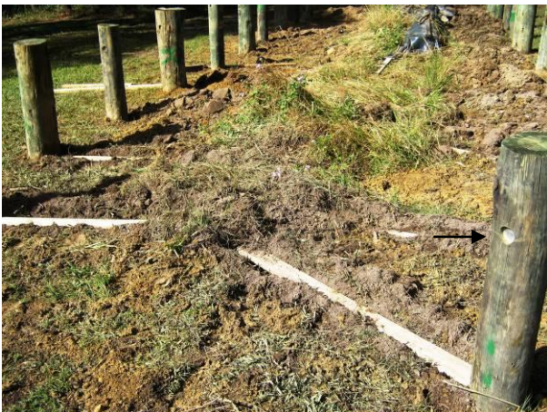
Figure 18 Feeder material connected to the trench
