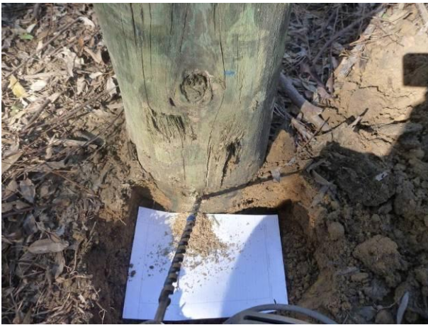
Figure 20 Drill shavings for examination
