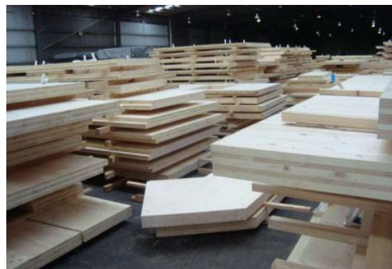
Figures 9 a and b The 10-storey ‘Forté’ apartment building in Bourke Street, Melbourne Docklands, under construction (2012); 760 CLT panels stored in a warehouse close to the site (source: Woodsolutions/C. Philpot, 2012; S. Lehmann, 2012)
