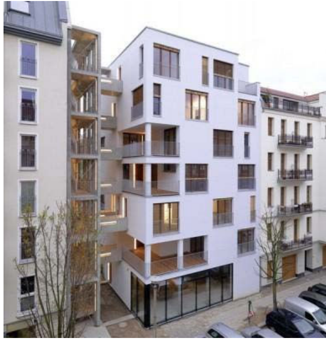
Figure 8. The 'e3' infill building, Esmarchstrasse, Berlin, a 7-storey residential urban infill building with a concrete staircase tower (source: architects)
