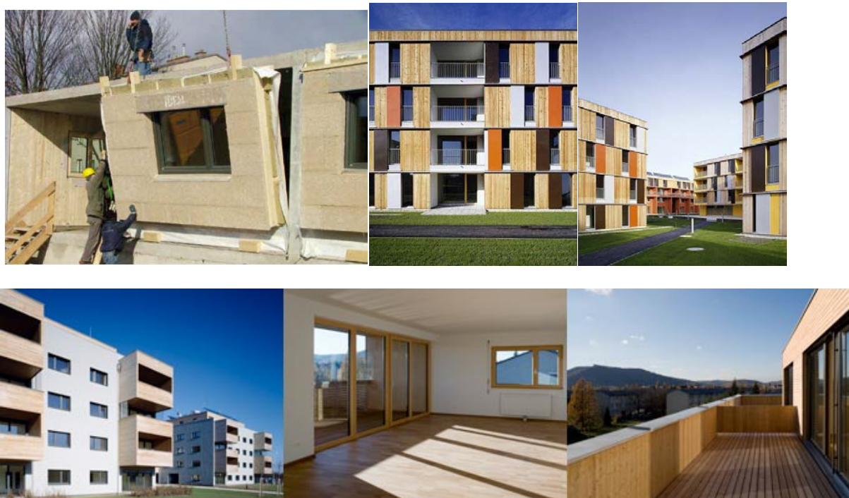
Figure 4 Images from Muehlweg project, Austria – exterior following completion, during construction showing prefabrication panels and interior ready for occupation (Source of images: http://www.trans-city.at/muehlweg.html )
