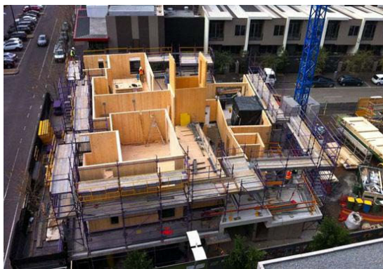
Figures 9 a and b The 10-storey ‘Forté’ apartment building in Bourke Street, Melbourne Docklands, under construction (2012); 760 CLT panels stored in a warehouse close to the site (source: Woodsolutions/C. Philpot, 2012; S. Lehmann, 2012)
