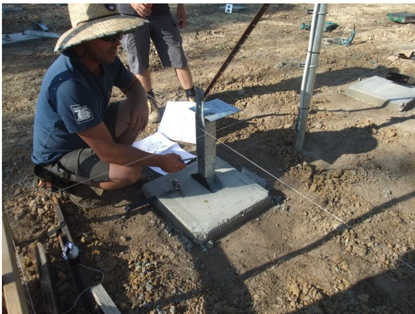
View across site showing footings and piers laid out
