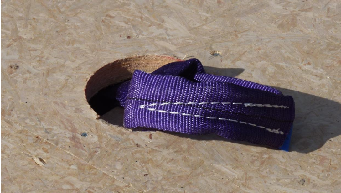
Photograph 5. Lifting sling positioned through hole in particleboard
