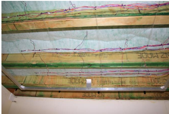
Figure 3. Floor frame from below with polyester insulation installed
