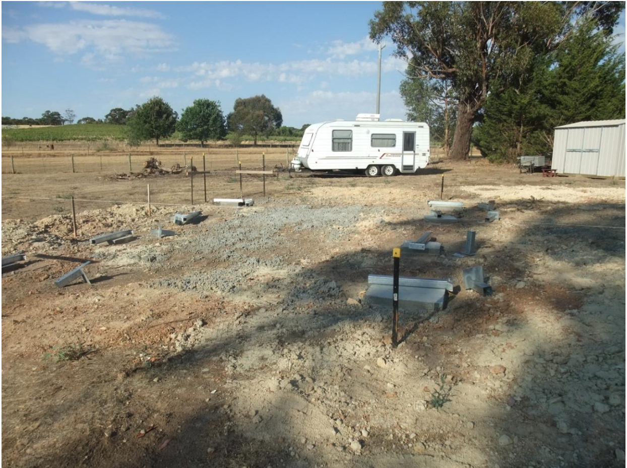
View across site showing footings and piers laid out
