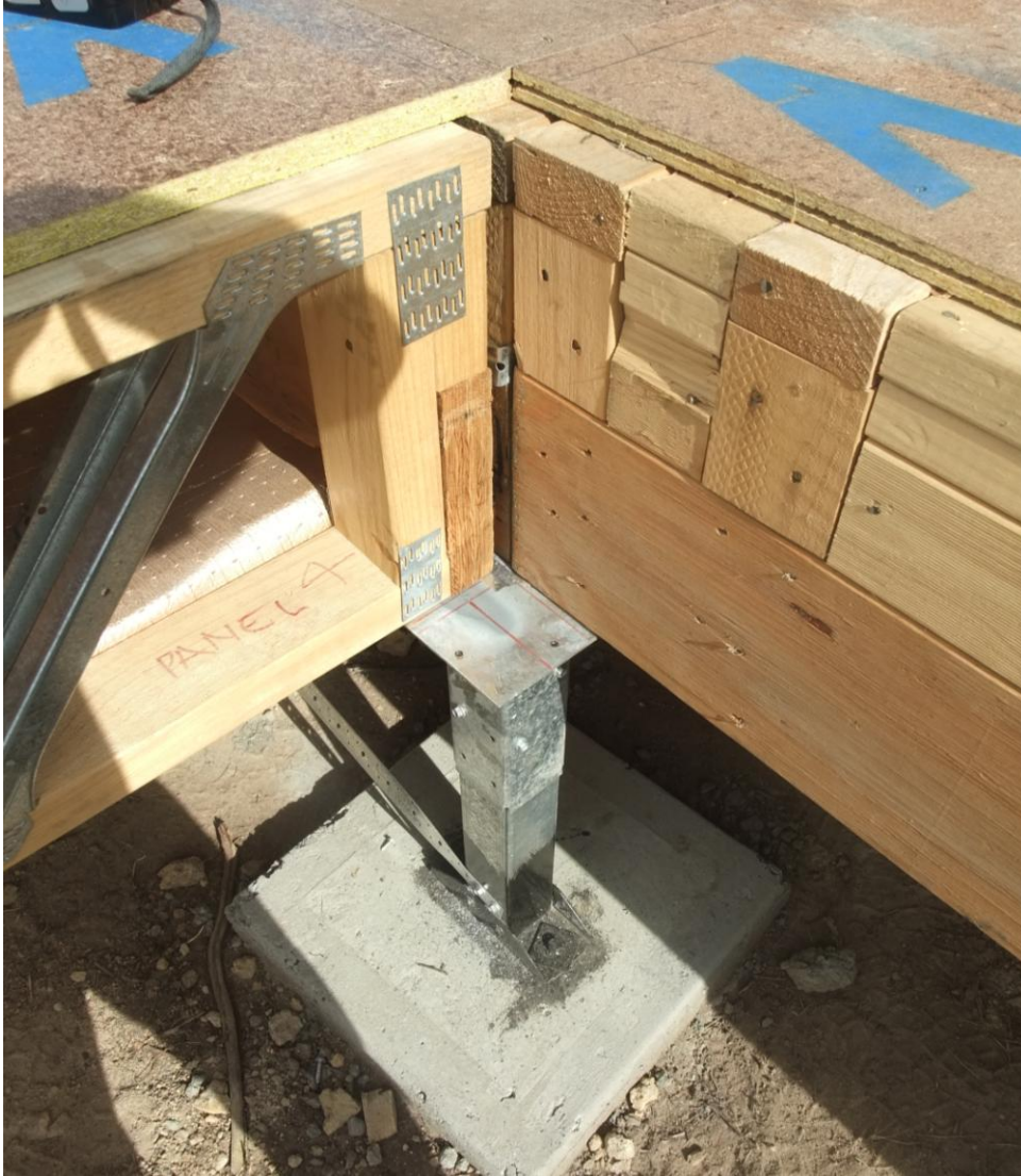
Detail of internal pier with three panels installed
