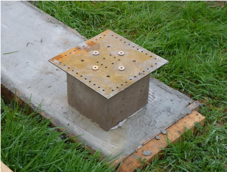
Photograph 3. Concrete support pier with connector plate
