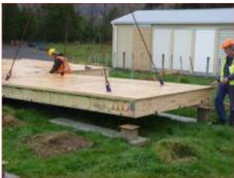
Panel lowered into position
