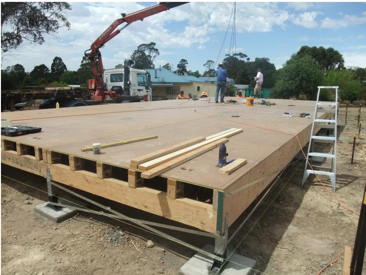
Floor with panels fully installed
