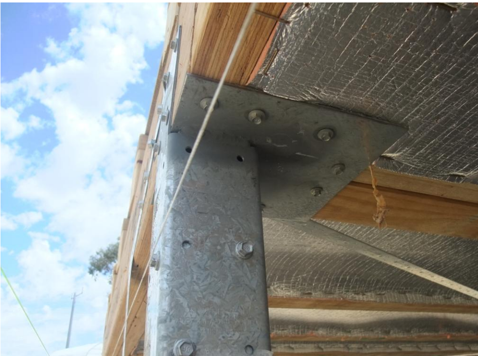
Detail of external pier with screw fixings
