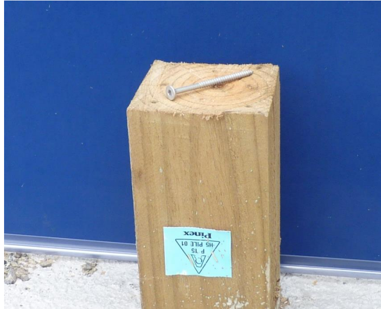
Figure 5. Timber stump with plate fixing screw
