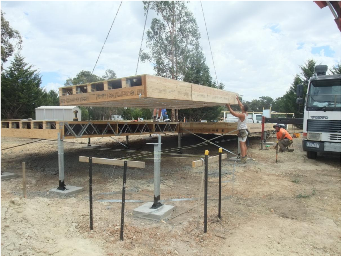
Installation of final panel (9)
