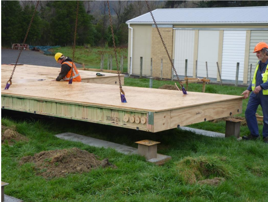
Photograph 6. Panel being lifted into position.
