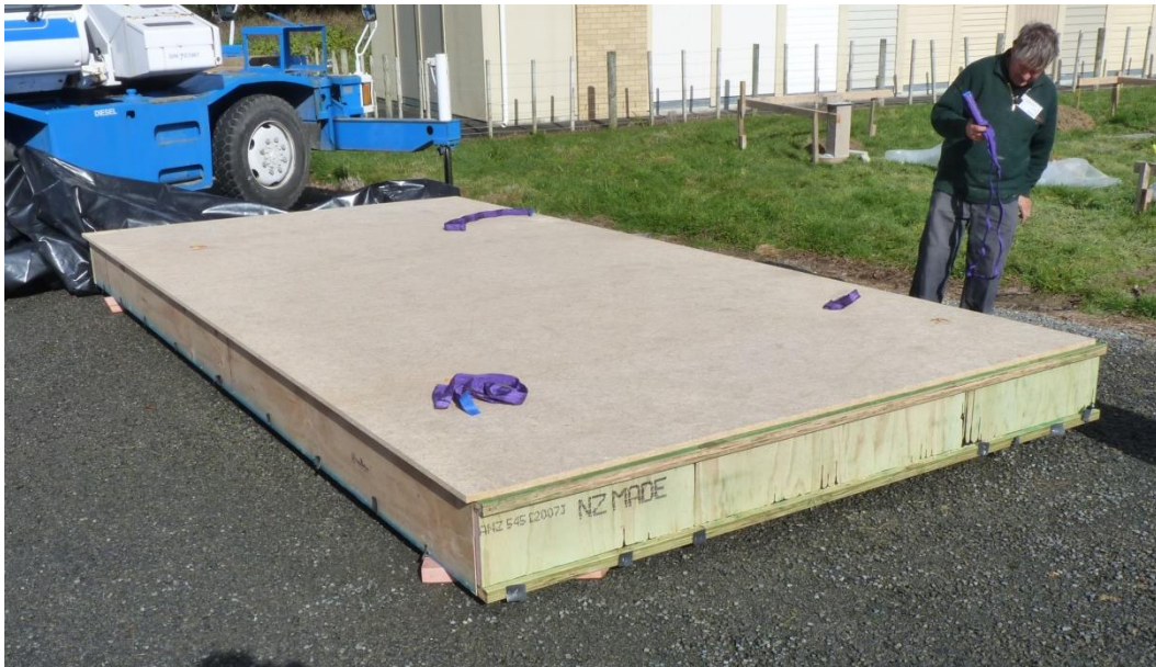
Photograph 1. Panel ready for erection. Lifting slings being inserted.
