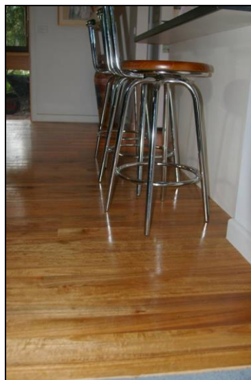
Figure 14: Corymbia spp. flooring produce from a kiln drying experiment with 10-22 year old pruned logs back-sawn at Auswest Timbers Pemberton, WA (Photo: Russell Washusen).
