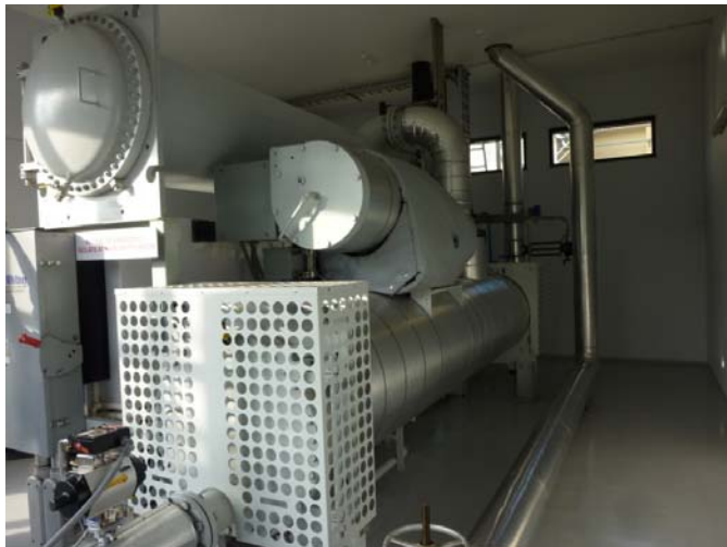
250 kW Purecycle unit at Gympie Timbers, Qld
