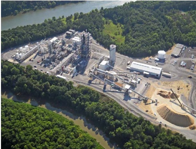
Figure 23 KiOR Mississippi plant 500 bone dry tons of biomass, to be completed in late 2012. (www.kior.com)
