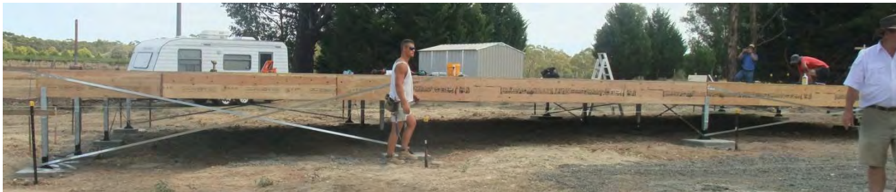
Floor panel site installation
