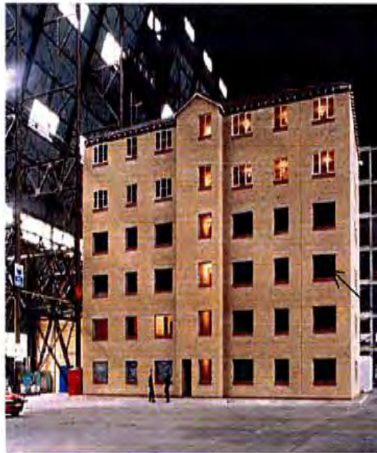
Figure 1: The six storey TF2000 building nearing completion situated inside Hangar No. 2 BRE Cardington.
