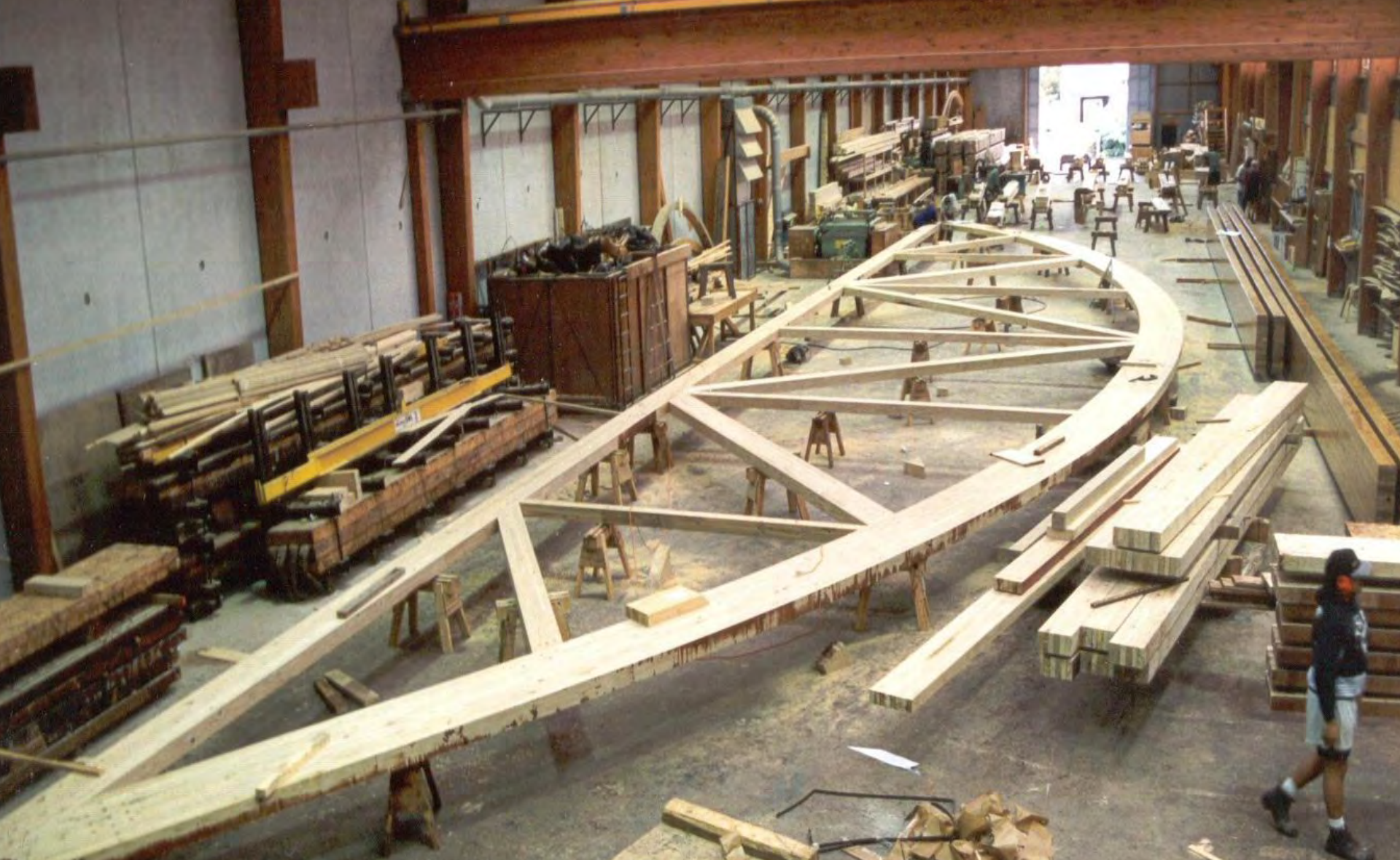
Main Structure – 34m Glulam Truss
