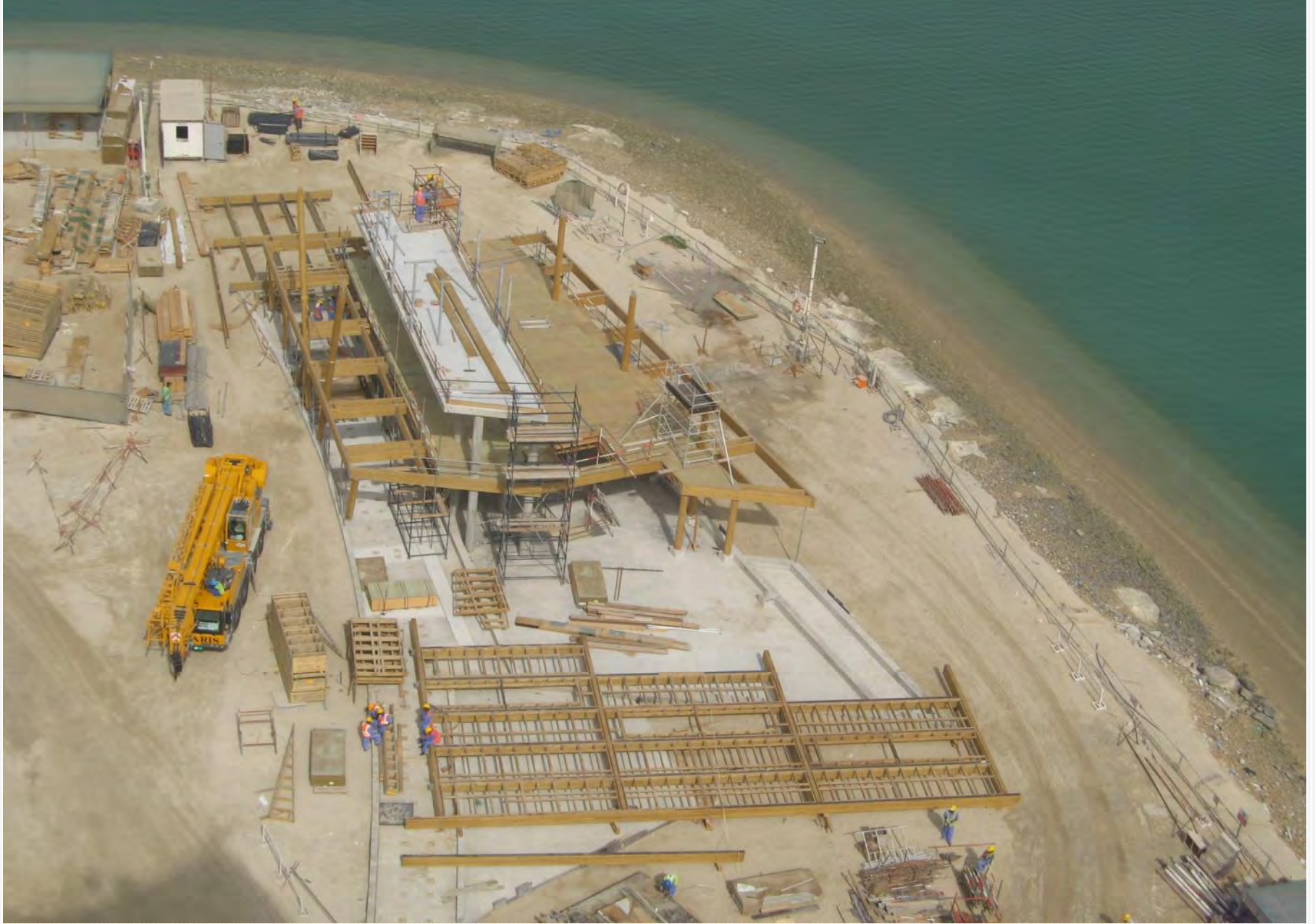
Roof Section Assembled on Ground
