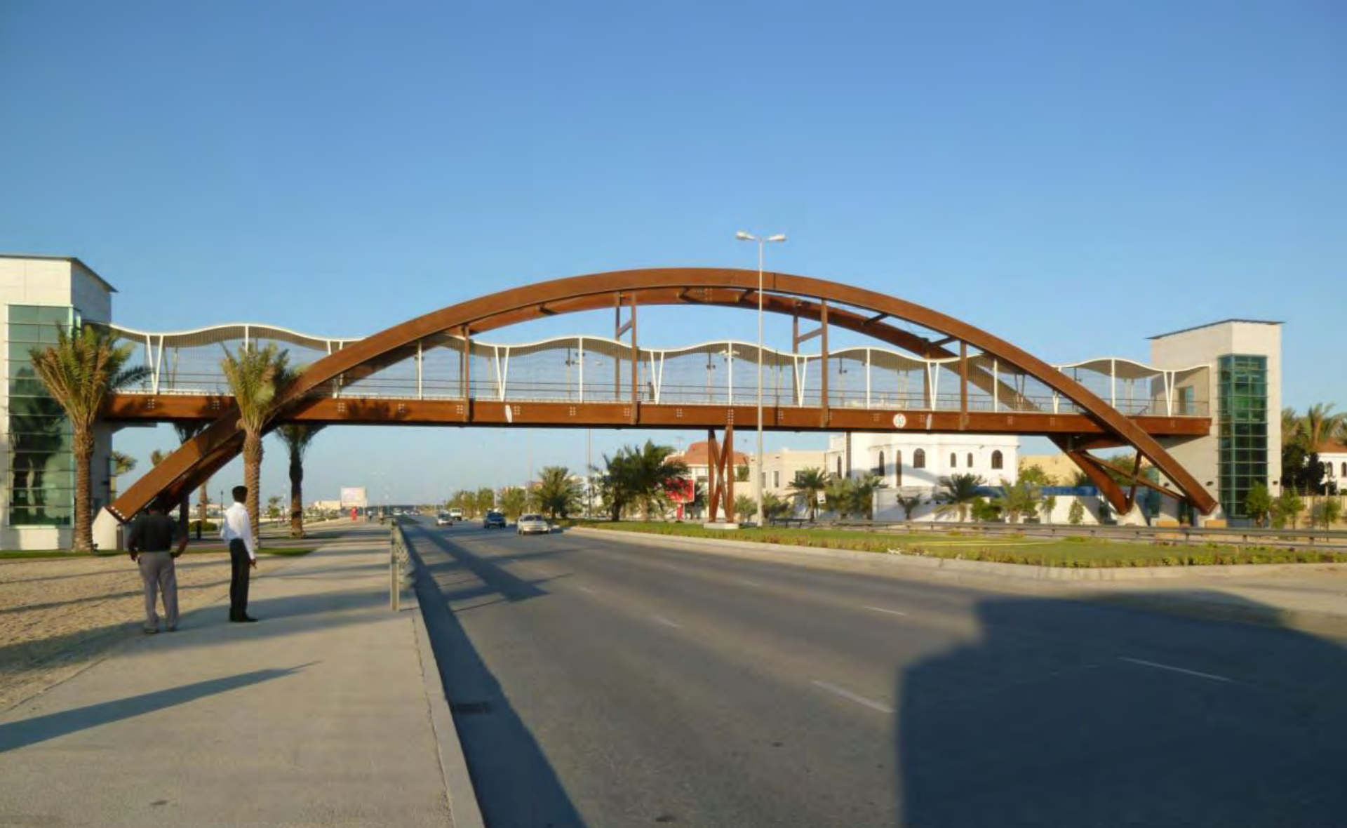
Pre Assembled Bridge – Installed over 5 nights – Minimal disturbance to traffic
