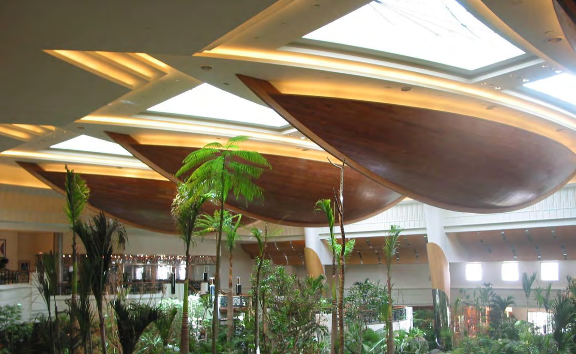
Finished Roof – 34m x 56m
