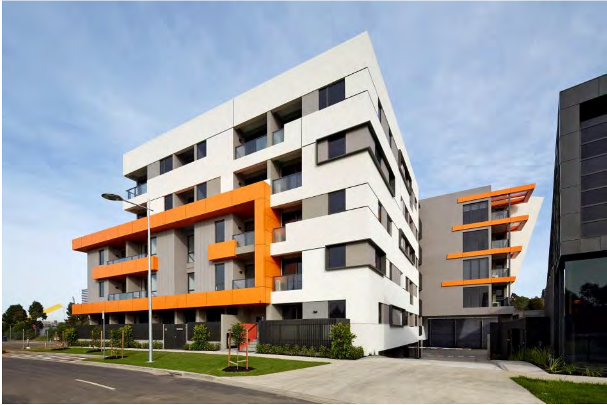
Figure 6 Study Building exterior.
