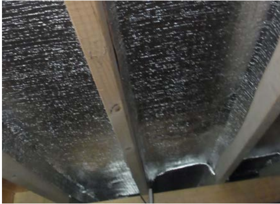
Figure 1: Industry installed reflective subfloor insulation
