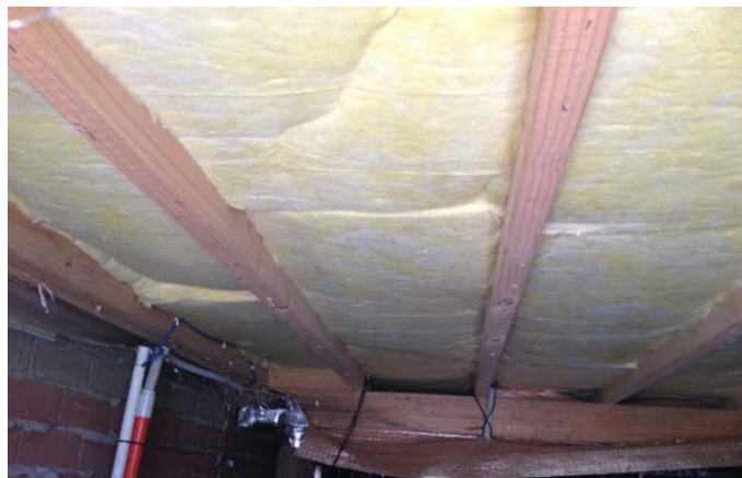
Figure 3: Industry installed bulk subfloor insulation
