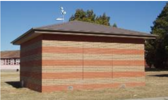
Figure 5: Enclosed-perimeter platform-floored test building
