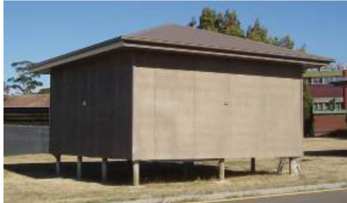
Figure 6: Unenclosed-perimeter platform-floored test building
