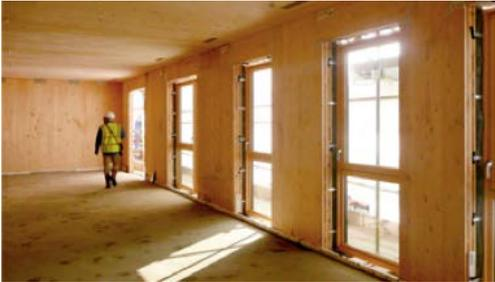
Figure 2: Photograph of CLT panel (Courtesy of Tilling)
