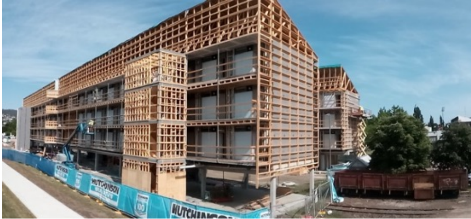
Figure 34. Nearing completion. All modules in place, CLT stairs, walkways and common areas installed, roof truss assembly completed and framing for external cladding completed. Image credit: CSAW
