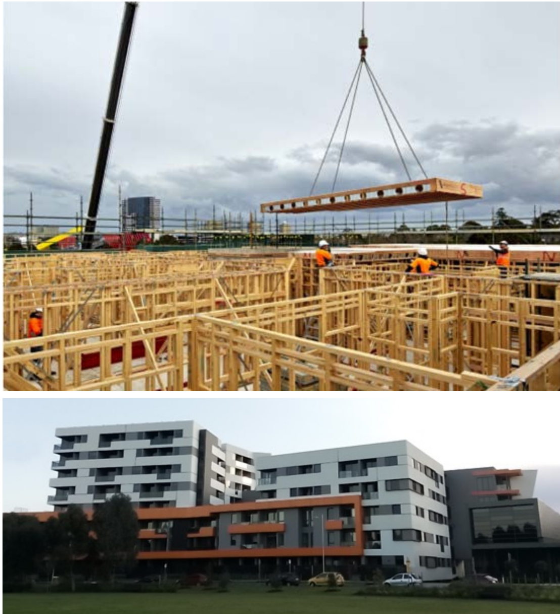
Figure 37. Top – Installing cassette flooring. Bottom – Completed building. Image credits: techbuild.com.au and D. Bylund
