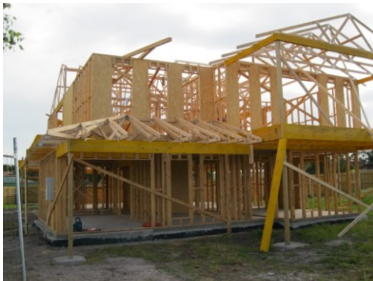
Figure 9 – A typical wall frame and nail plated roof truss house under construction in Australia. Image credit: CSAW
