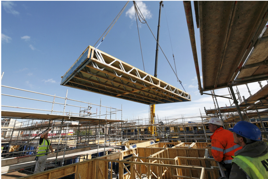
Figure 31. Hybrid timber steel cassette floor being lowered into position Image credit: Unknown
