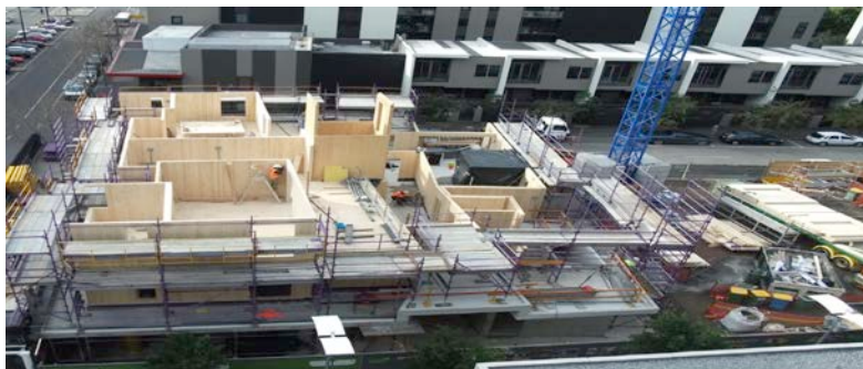
Figure 23. CLT installation at the Forte Living project, Docklands Melbourne. Note the proximity to occupied apartments to top of image, also limited impact: small on-site staff, small remote control crane, one truck movement per day with CLT panels.
