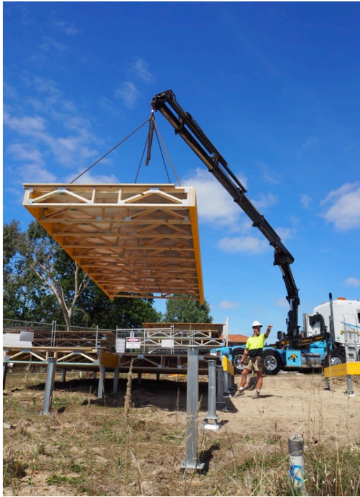
10a Ground floor cassette system on a Surefoot non-concrete footing system
