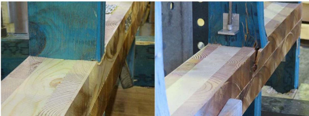
Figure 33: Indenting and Spiriting of CLT Wall
