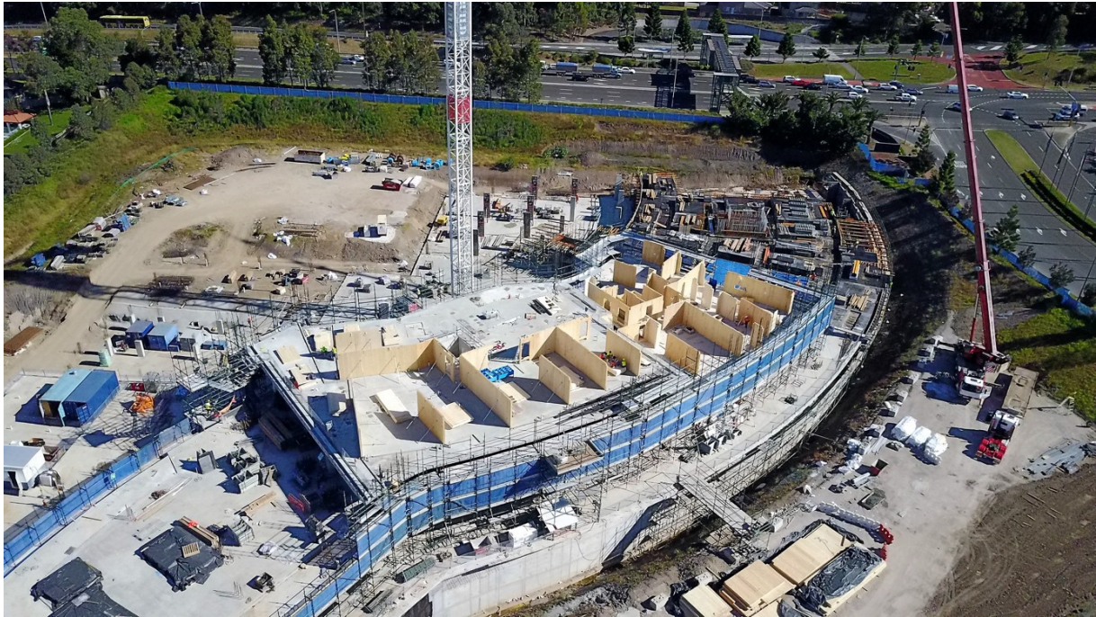
Figure 9: CLT Construction site with staging area (lower right)
