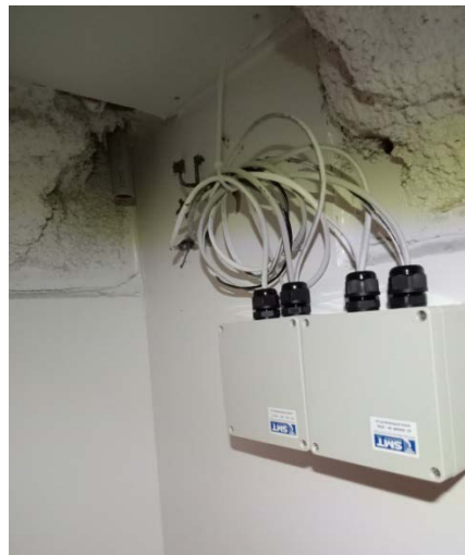
Figure 24: PMM wires penetrating wall in the garbage room and connected to A3 Data Acquisition Units, Image Credit, TDA
