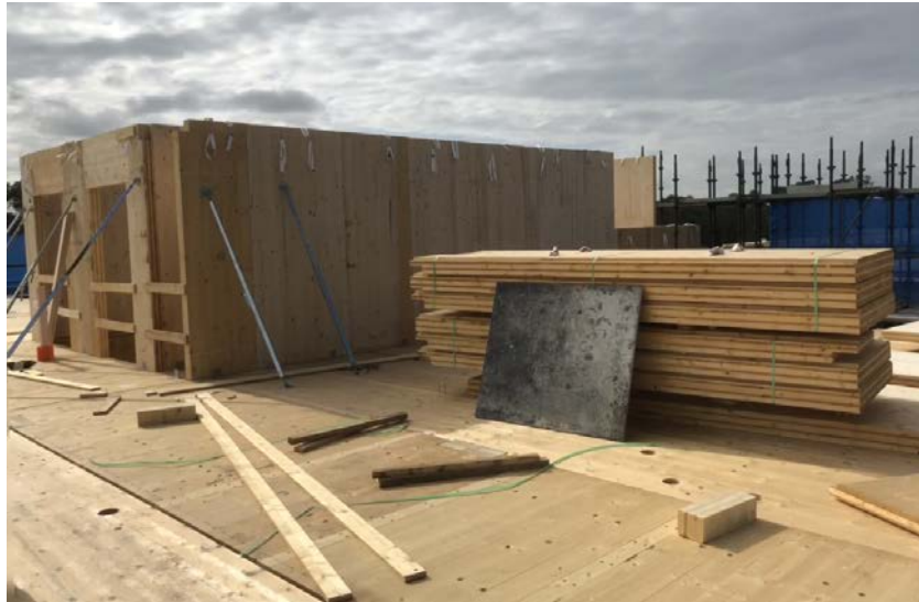
Figure 4: CLT floor and lift core at Phoenix, Image Credit: TDA
