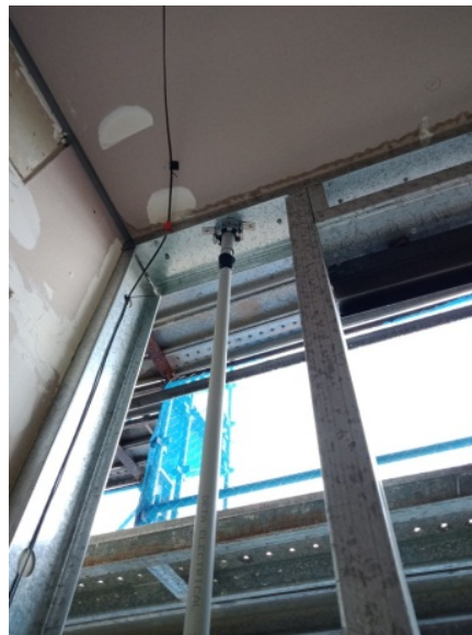
Figure 17: 25 and 32 mm conduit in a wall cavity with fire-rated collar, Image Credit: TDA
