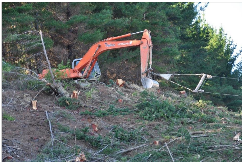
Figure 16: Excavator being used as a mobile tailhold. (Photo: P. Millikan / ATL).
