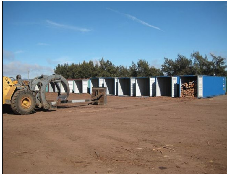
Figure 5. A detachable pusher plate that is held in the forks of a rubber-tired loader and used to push protruding logs into a container.
