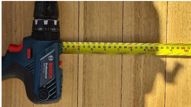
Figure 4: Regular gapping in floor
