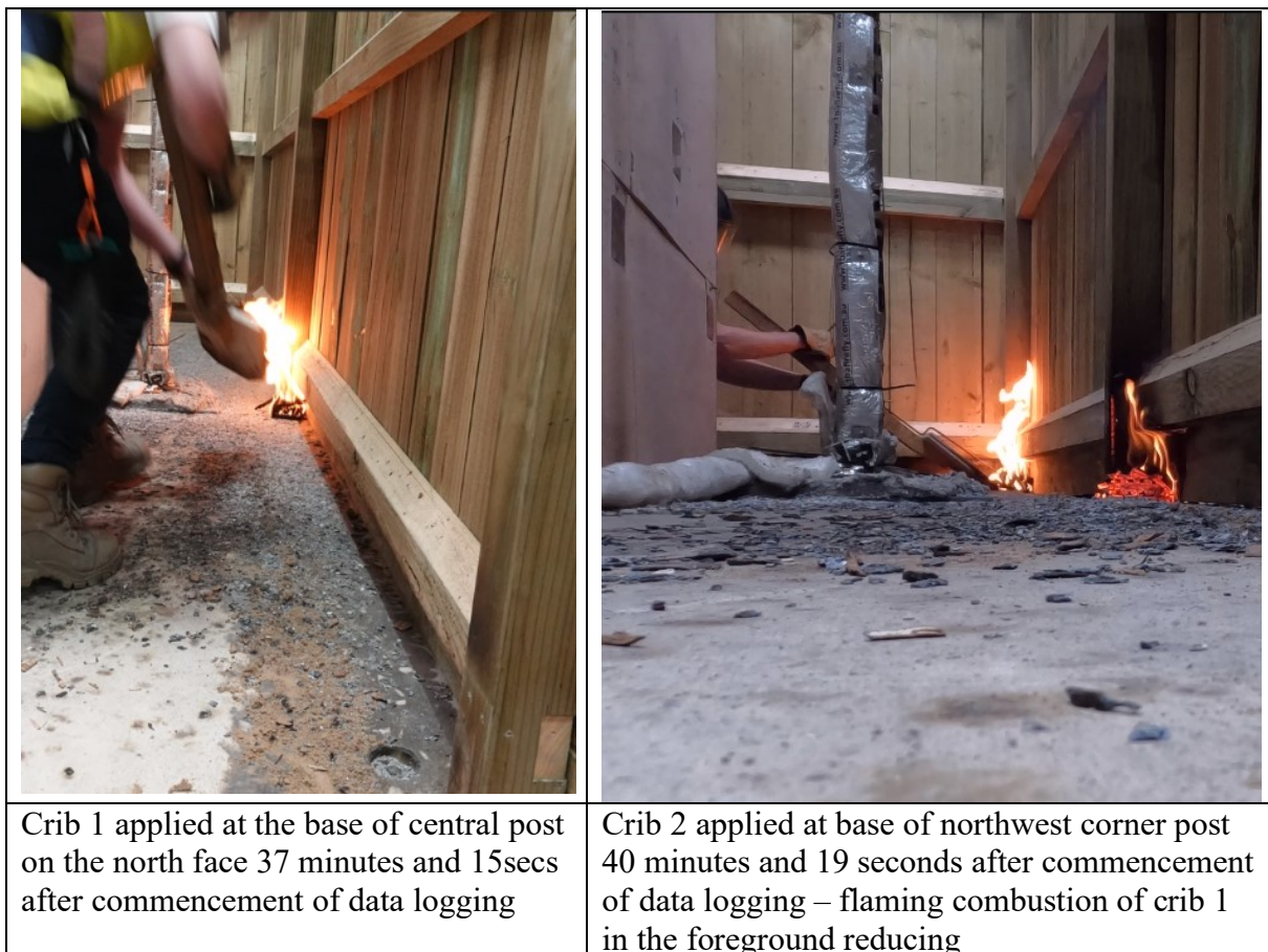
Figure 81 Placement of timber cribs.
