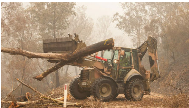
Figure 18: Excavators and backhoes
