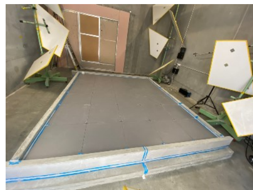
(b) Two rows of horizontally laid perimeter concrete sleepers plus a row of vertical sleepers
