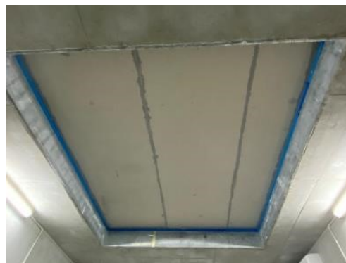
Ceiling with Acoustic Sealant Treatment
