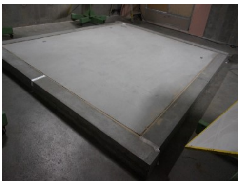
(a) Two rows of horizontally laid perimeter concrete sleepers
