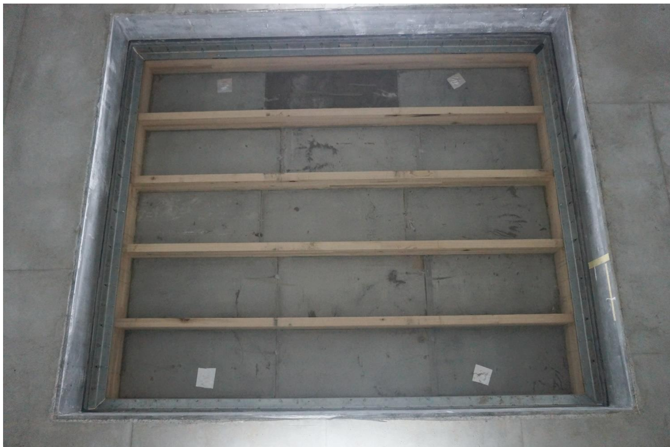
Underside of ATC Composite Panel, installed in laboratory resting on steel ledge (as tested)
