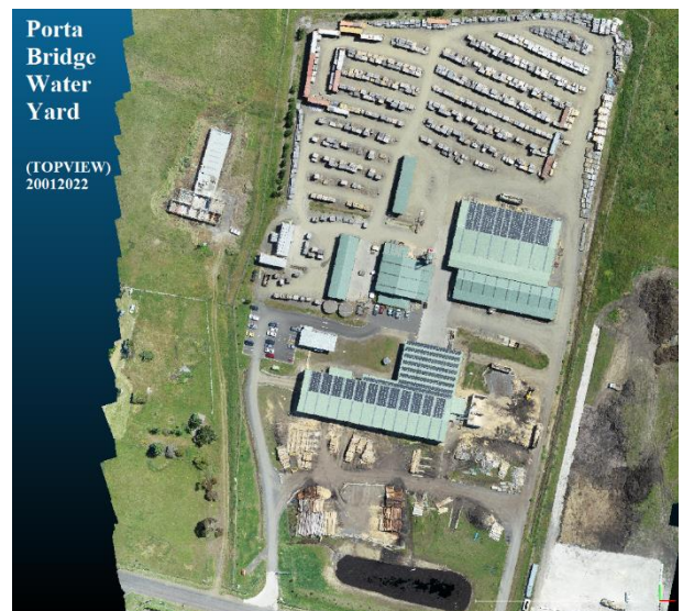
Porta Mouldings Bridgewater drying yard
