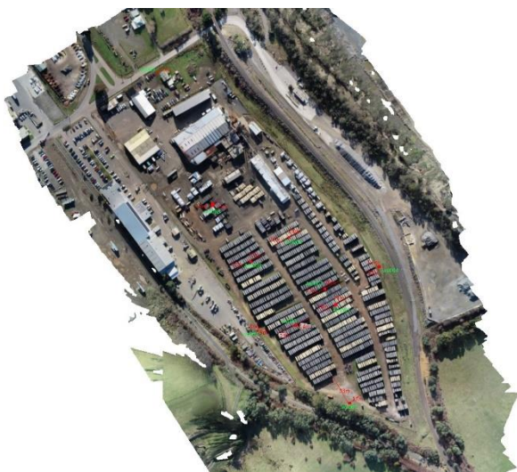
NSFP's Mowbray drying yard
