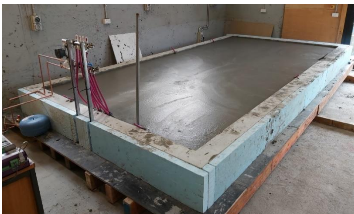
Figure 25: Topping to the heater slab
