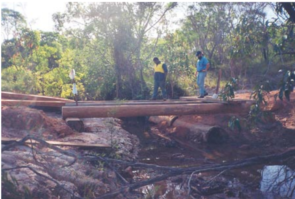
Figure 18: Sustainable native forest management at Injinoo community allows local native forest timbers to be used for bridge construction.
