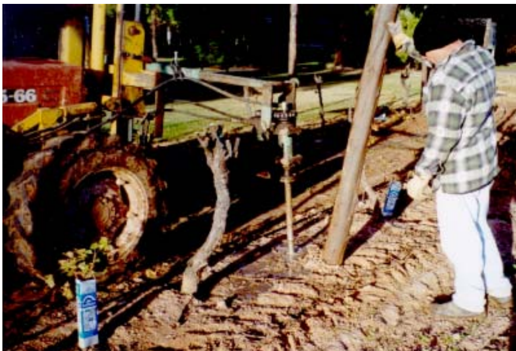
Figure 19. Trellis post hole being drilled and water squirted into hole to create a slurry
