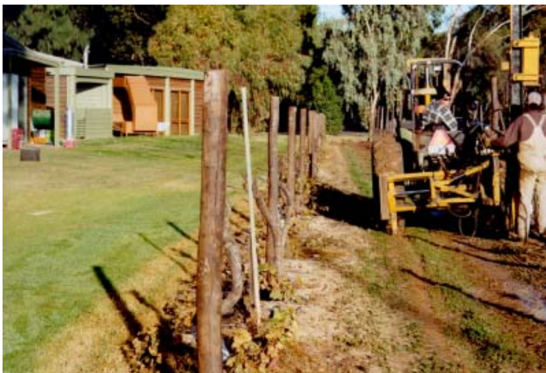
Figure 21. First row of PEC-treated posts next to the wine tasting and sales area at Southcorp (Lindemans) winery.
