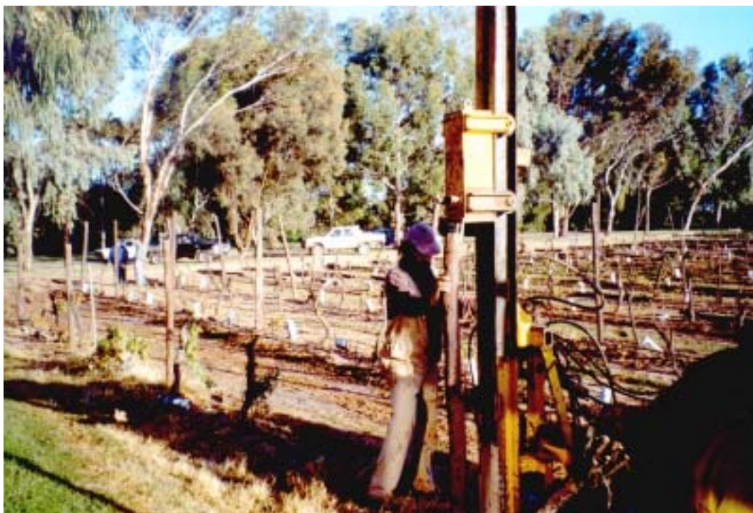
Figure 20. Eucalypt trellis post being rammed into position
