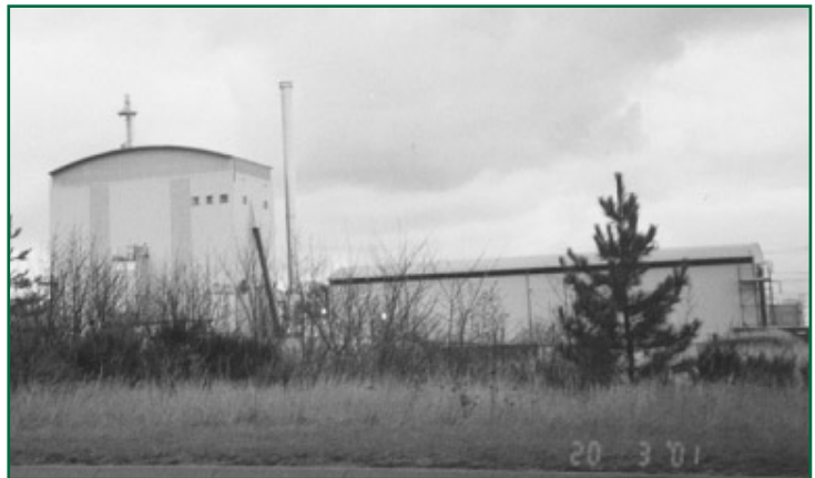
Figure 1. ARBRE 10 MW power station in Leeds, UK using new gasification technology with combined cycle gas turbine and steam turbine electricity generation. Short rotation intensive culture coppicing willows will be used for fuel. The project is currently being commissioned.
