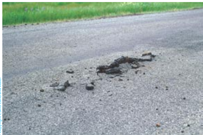
Example of road damage near Griffith NSW caused by high water table levels and salinity.
