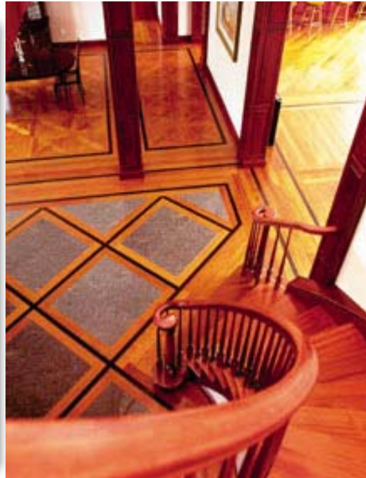
Feature flooring showing inlays
