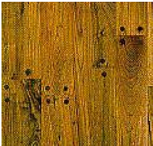
Scerri plank floor plugged
